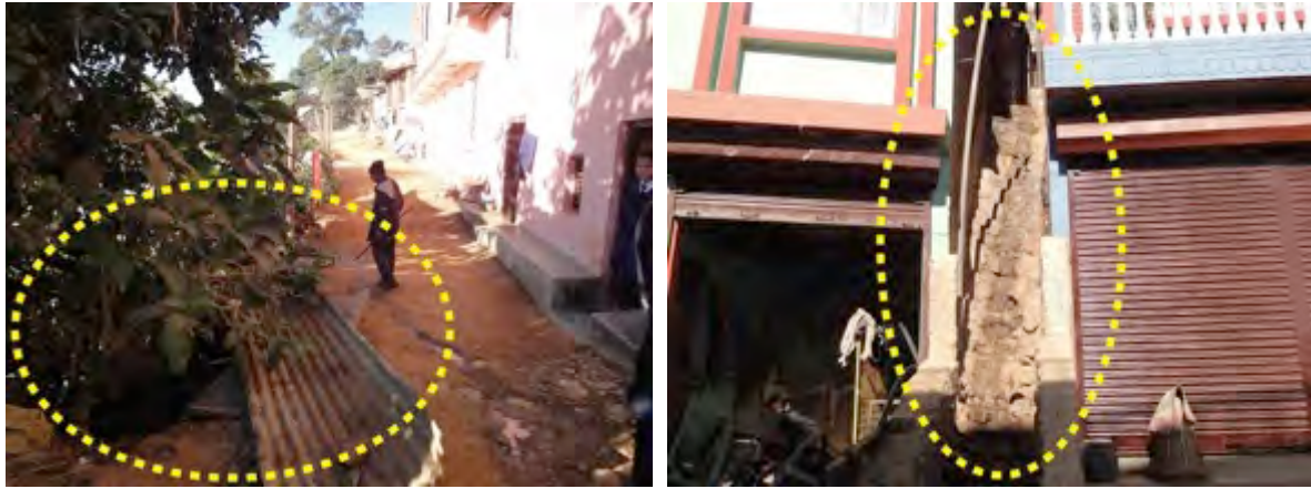
Figure 27: A blocked sewerage drain causes wastewater to pool along the main thoroughfare and trickle downhill past the houses located below (Bright-Davies).
