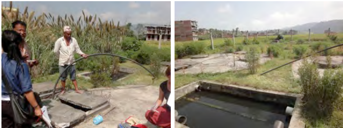
Figure 18: Photos of the constructed wetlands and biogas chambers at Srihandapur, with on-site caretaker (Bright-Davies 03.10.12)
