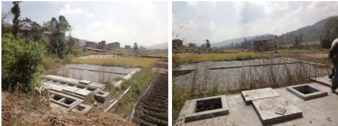
Figure 22: Photos of the ABR and horizontal flow, gravel-bed filter in Nala (Bright-Davies 17.10.12)
