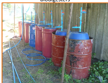
Floating drum gas reservoirs at the Royal University of Agriculture
