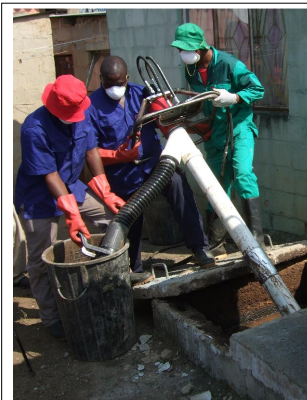
Fig. 3. Extraction auger in use in Durban, SA.
