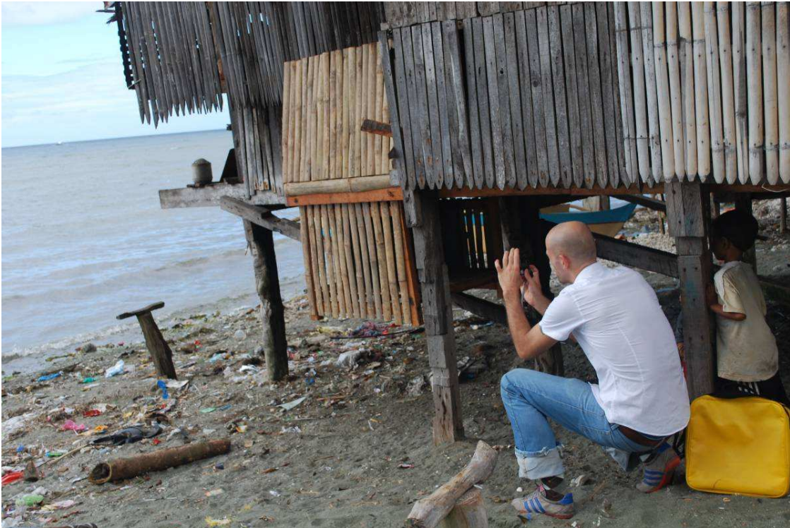
Photo 2. View of a classic “hanging” ecosan toilet. The upper portion is the toilet while the lower portion is the container that stores the faecal matter and urine. Tidal waters do not affect the toilet.
