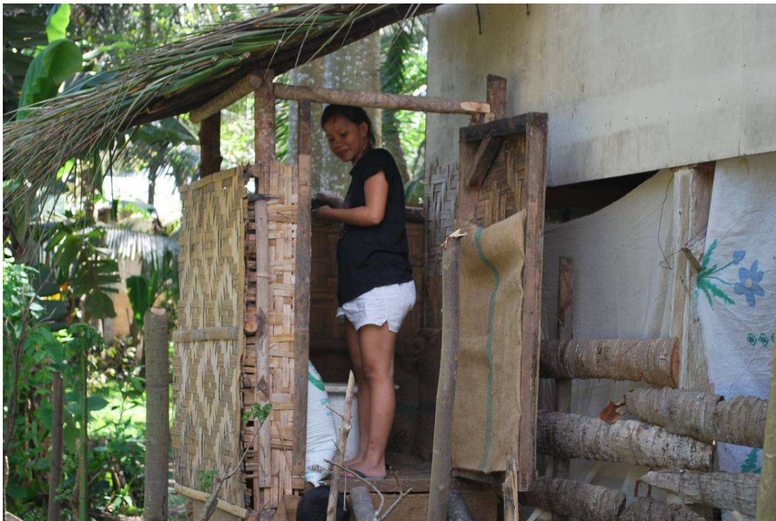
Photo 1. Simple ecosan toilet built beside a house. The materials comprising woven coconut palm fronds for roofing, woven bamboo slats, round wood poles, coconut lumber are all locally procured. Local people here are expert bamboo and palm weavers.
