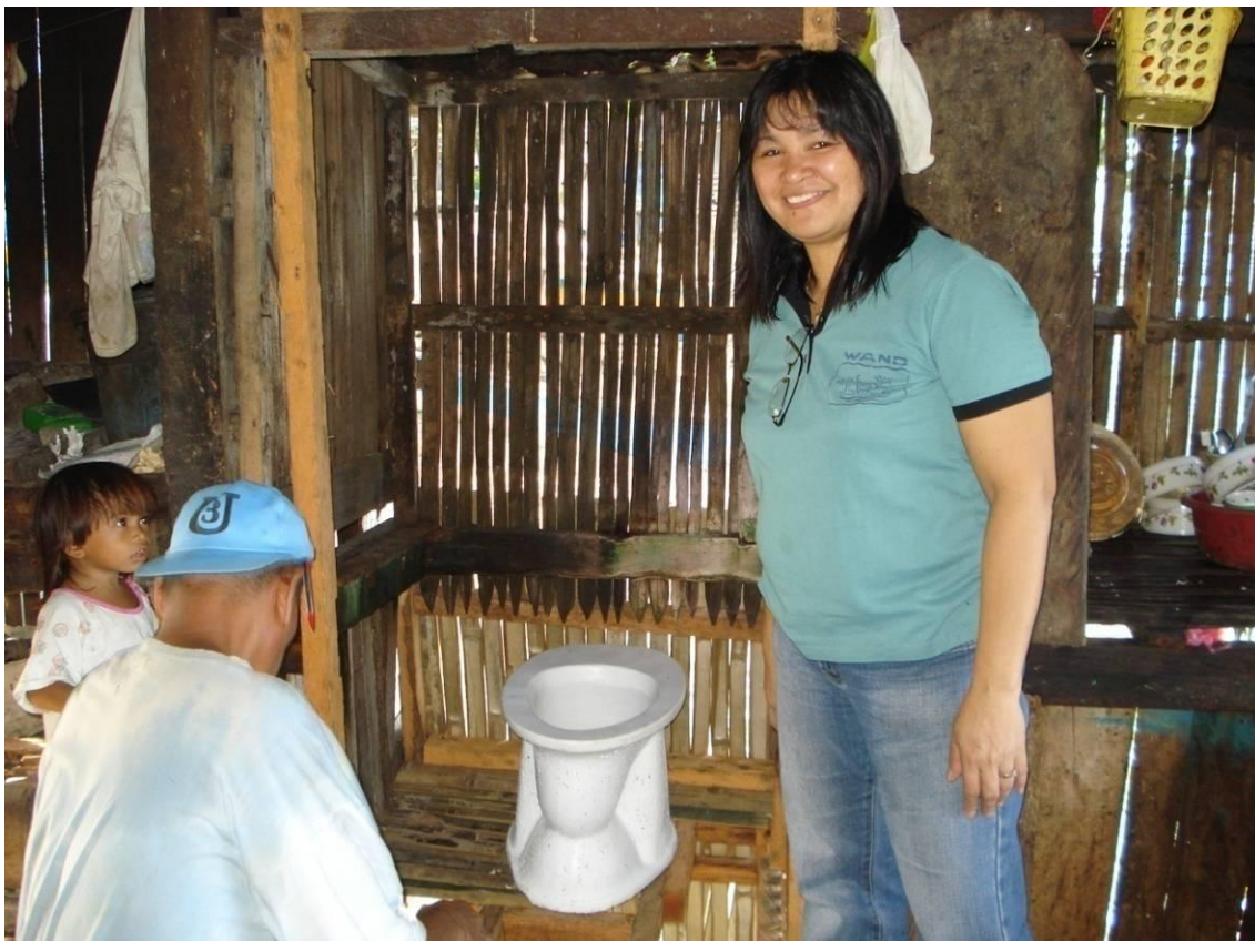
Photo 15: Inside view of a coastal ecosan toilet. The toilet is built at a side of the house
