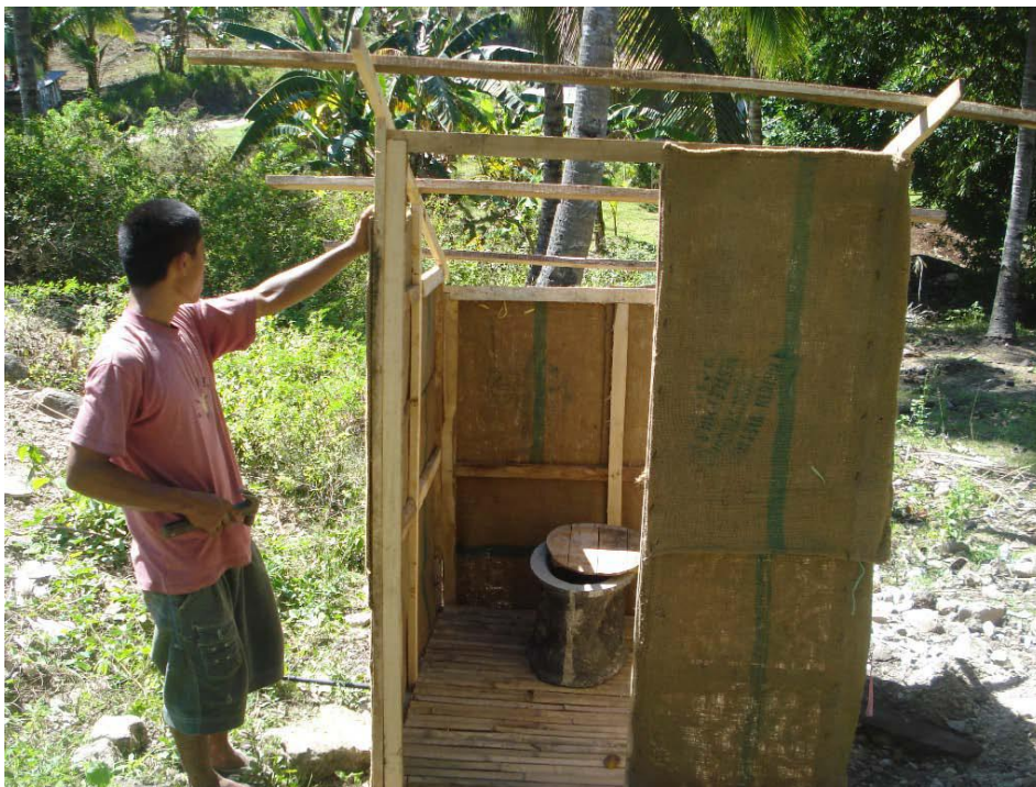
Photo 27: A beneficiary helping construct his arborloo ecosan toilet.
