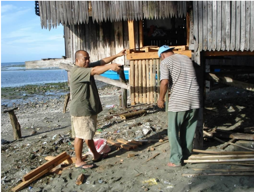
Photo 28: The author supervising the construction of a hanging ecosan toilet.
