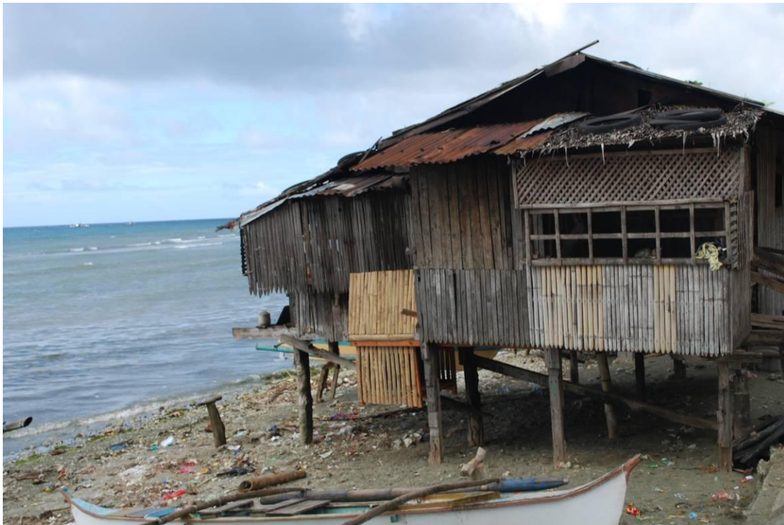
Photo 16: The house showing the view of the hanging ecosan toilet, Initao Municipality.
