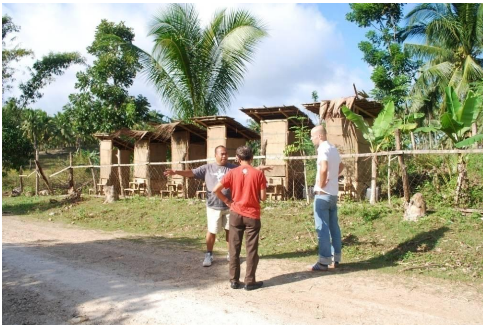
Photo 14: Single-vault ecosan toilets lined-up for transport. The beauty of this system is that this can be used as emergency toilets during situation of mass evacuation and
