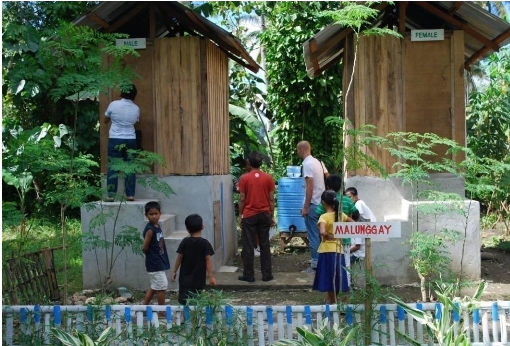
Photo 7: Two double-vault ecosan toilets located in Tuod Elementary School, Manticao, Misamis Oriental. Urine fertilizer is used by the school children in the vegetable and flowers surrounding the school.
