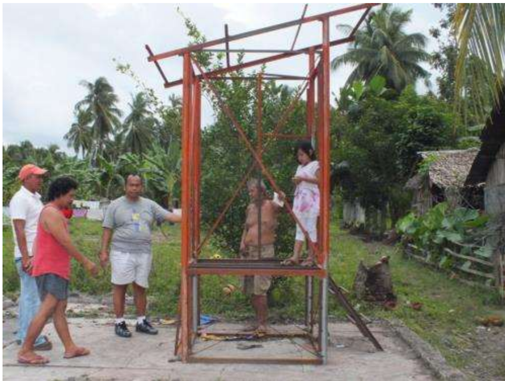
Photo 6. Steel-frame for a single-vault ecosan toilet.
