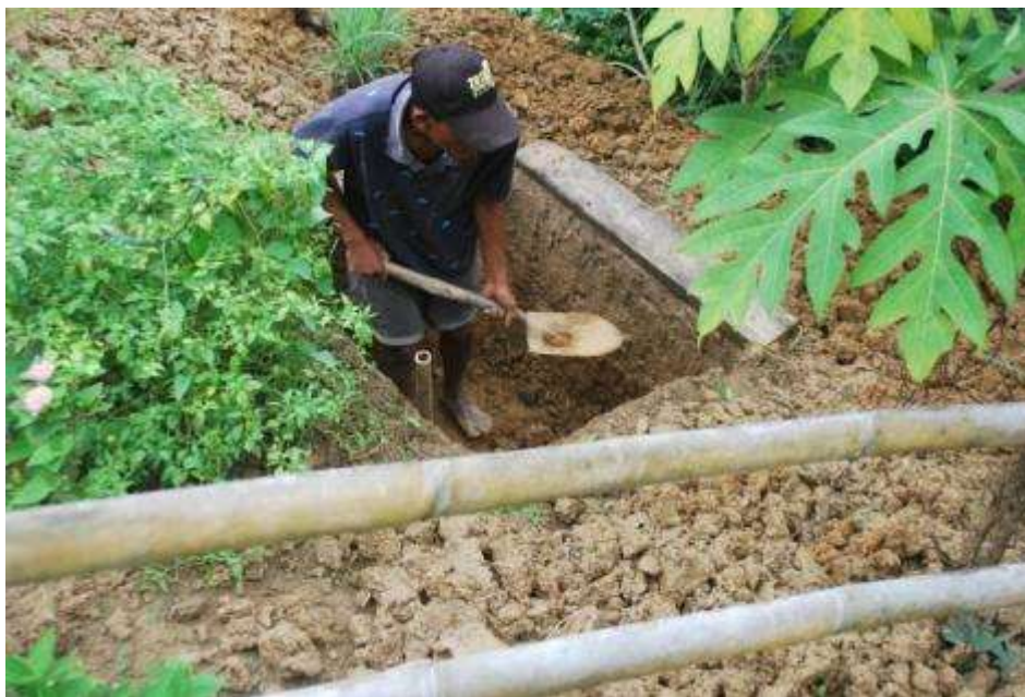
Photo 10. Preparing the pit for the arborloo toilet.
