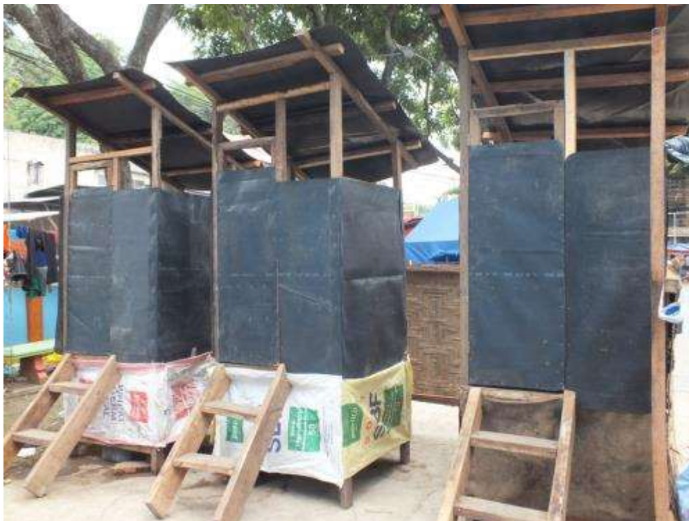
Photo 3. Ecosan toilet made of recycled materials.
