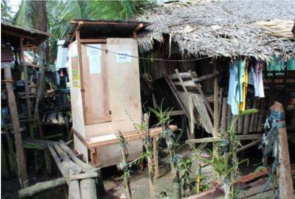
Photo 4. Single-vault ecosan toilet in a flooded zone.
