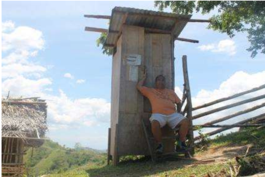
Photo 9. Single-vault ecosan toilet in a mountain area. This is not suited in hillsides where strong wind can easily topple the structure.
