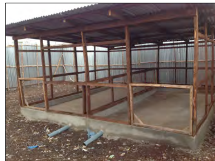
Figure 13 Compost Bay, May 2013
