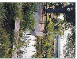
The wetpark in Kalmar, Sweden Greywater is purified to potable water quality. The greywater from the technical high school is purified in a series of ponds, using the same principles as the living wall. An excess of 700 m 3 water of potable water quality is attained each year.
