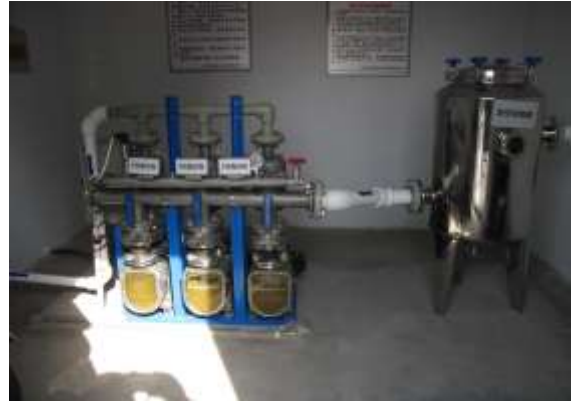
Figure 5 vacuum pump-unit and buffering vessel
