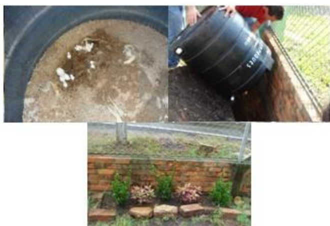
Fig. 10: Treatment and final productive disposal of treated fecal matter. La Horqueta school. (Photos: Gutiérrez and Rodríguez 2012)
