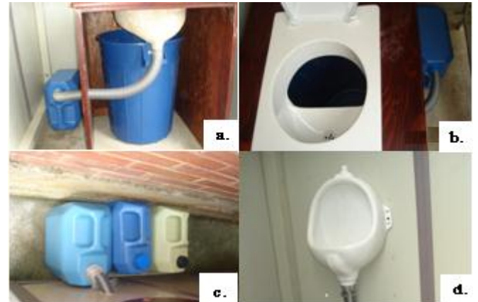
Fig. 8: Model 2: a) urine and fecal matter collection tank; UDDT seat; b) urine collection tank; c); and d) urinal (Photos: Gutiérrez and Rodríguez 2011)
