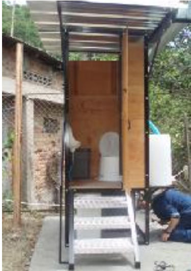
Fig. 5: Prefabricated UDDT unit, La Horqueta school, Model 1. (Photo: Gutiérrez and Rodríguez 2011)
