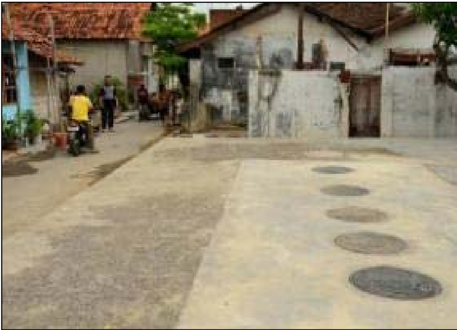
A communal wastewater treatment plant serving a simplified sewer network in east Tegal, Indonesia.
