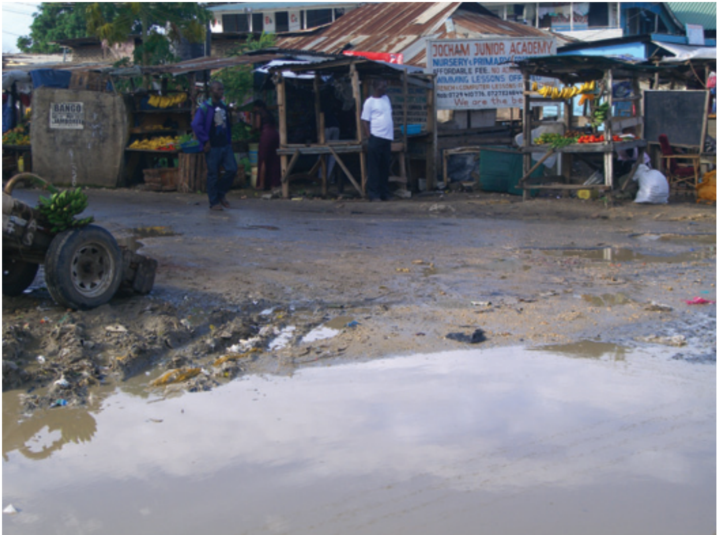
Inadequate drainage in a peri-urban neighborhood of Mombasa, Kenya.
