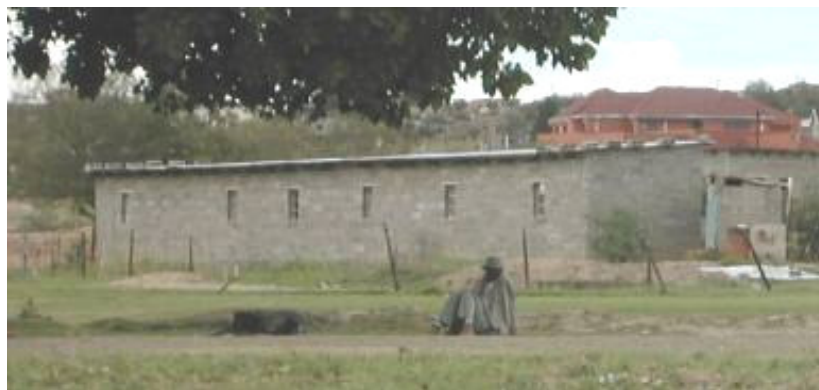
Maleane rental house in Maseru. It is likely that 6 or more rooms are rented out to separate groups and they share the VIP.
