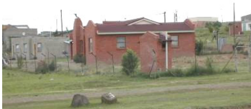
Brick VIP in foreground where roof tiles match those of the house behind. This 'customisation' of VIPs in Maseru is not uncommon – reflecting the 'status' marketing VIPs.
