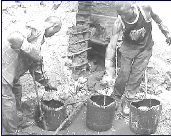
This Nairobi latrine is not rebuilt when full. The pit sludge is removed manually (and dumped round the corner). © Sabine Bongsi / WSP
