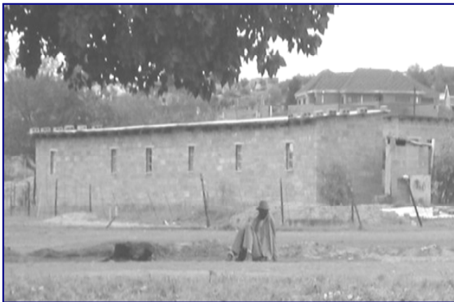
A Maseru line house of rental rooms with shared latrine
