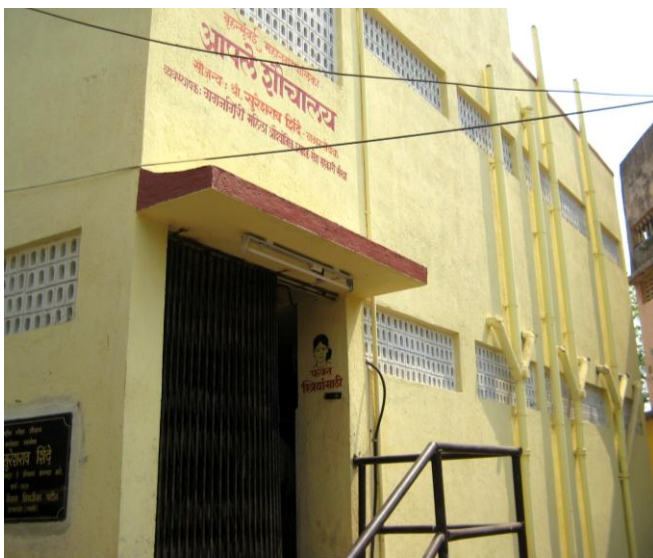
Fig. 5: New community toilet block constructed under the SSP with separate entrances for women and men in order to enhance private sphere and security for the women (source: Keller 2009)
