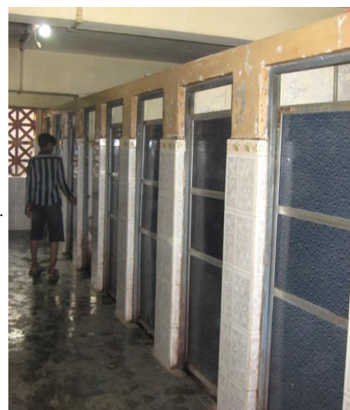
Fig. 6: Community toilet block constructed under SSP with a number of 20 toilet seats, located in Govandi slum (source: Keller 2009)
