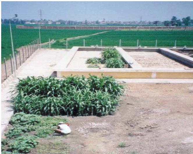
Fig. 5: Conversion work in Nawaq (source: IPP)
