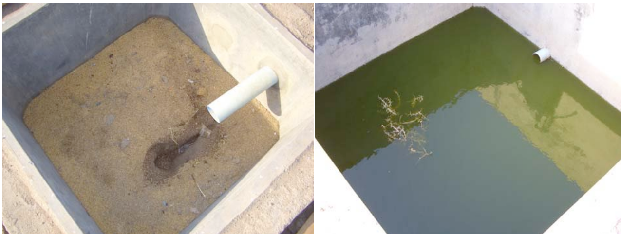
figure 18: Vertical flow organic filter (left) and collection tank for greywater (right)
