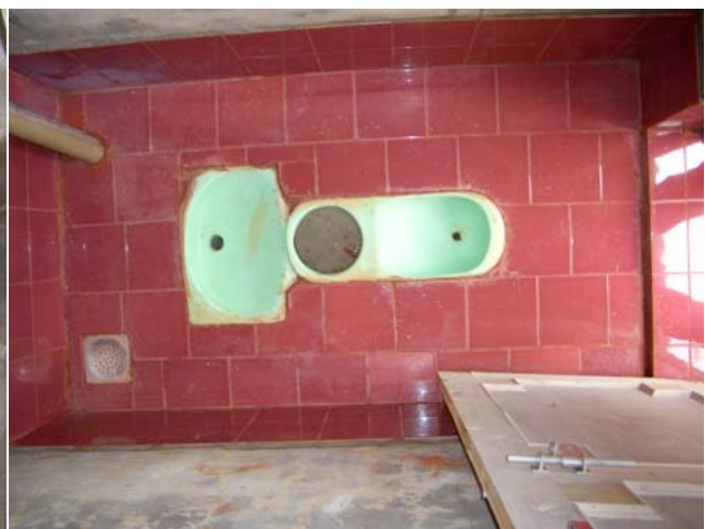
figure 11: Urine-Diversion Dehydration Toilet [clockwise from top left: view of Urine-Diversion Dehydration Toilet designed by a team from the Massachusetts Institute of Technology; view of squatting pan that allows source-separate collection of urine, feces and cleansing water; top view of toilet cubicle; view of piping system below squatting slab]
