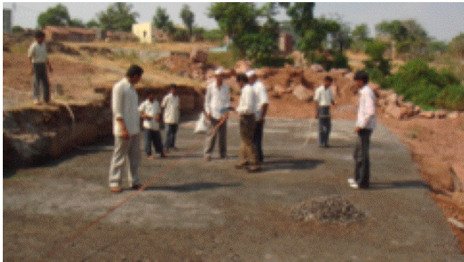
Fig 5: Horizontal Flow Constructed Wetland for...? (under construction) Where...? Month, year? (photo: N. Zimmermann)
