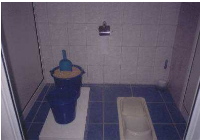
Fig. 9: Ecosan UDD toilet interior. On the left: squatting pan covered with lid and bucket with sawdust. On the right: squatting pan in use (source: AWHEE, 2006)
