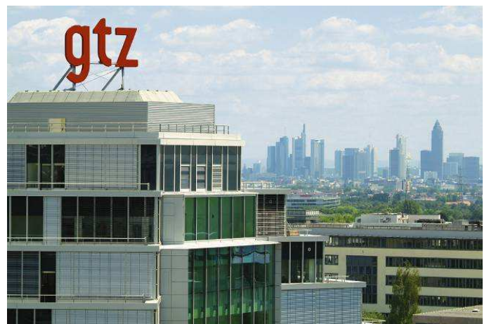
Fig. 3: The main building ("House 1") at the GTZ headquarters in Eschborn near Frankfurt, where this project is implemented (source: GTZ).
