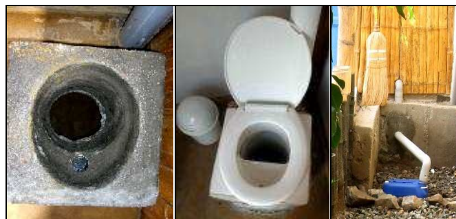
Fig. 12: Toilet seats without (left) and with (middle) plastic insert for urine separation. Pipe from UDD toilet to 25 L urine jerrican (right).
