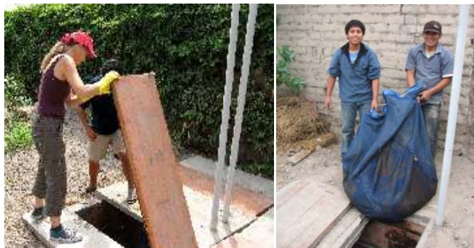
Fig. 6: Double-chamber compost filter ("Rottebehälter") for blackwater pre-treatment (left) and removal of a filter bag (right)
