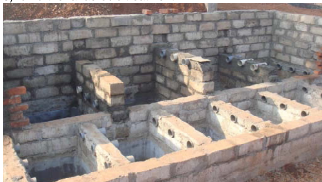
Fig 5: Construction of ABR and UF (photo: N. Zimmermann)
