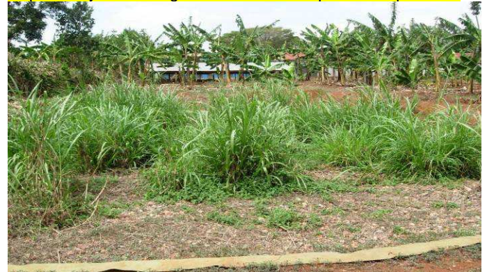
Fig. 8: Constructed wetland, planted with xxx (source: EcoSan Club, year?)
