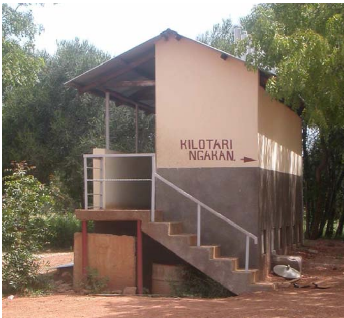
Fig. 5: New "compost" pit latrines for patients after reconstruction, side view (source: EcoSan Club, 2004)
