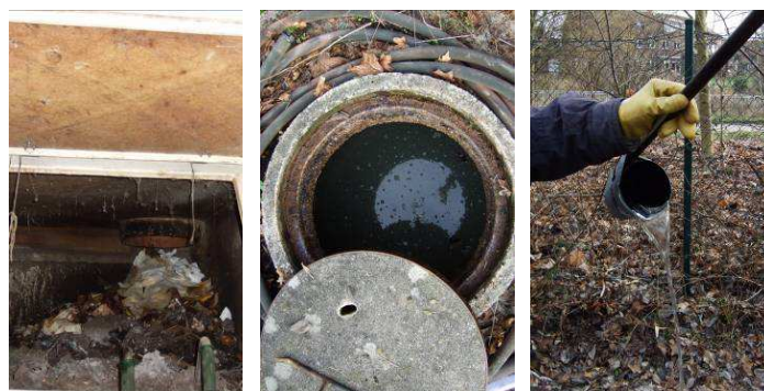
Fig. 10: Compost heap inside the composting container of the toilet (left), greywater in Imhoff tank (middle) and final effluent from constructed wetland (right). Source: A. Schöpe, 2009.
