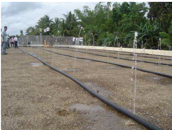
Fig. 7: Testing distribution system of wastewater on vertical soil filter (cell 1 of constructed wetland), June 2006 (source: DILG-GTZ Program).
