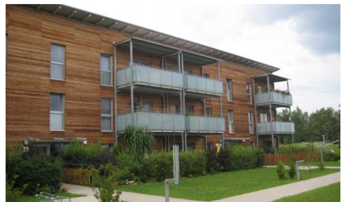
Fig. 3: Buildings of the ecosan project in solarCity (source: Hochedlinger, LINZ AG, August 2009)
