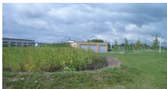
Fig. 9: Constructed wetland (reed beds) in operation (source: LINZ AG, May 2008).
