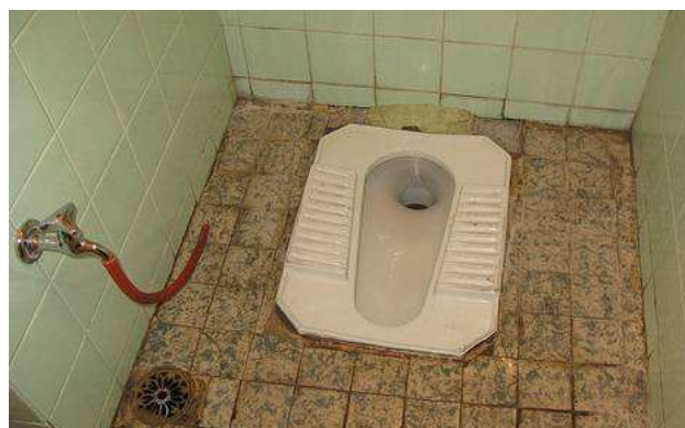
Fig. 5: Typical toilet in Syria: Squatting type with flushing. Hose on the left is for anal washing with water. Source: E. v. Münch, Jan. 2009.
