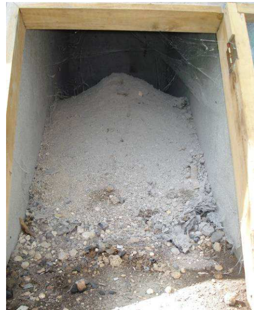
Fig. 10 Inside view of a faeces vault (with faeces and ash) of a double-vault UDD toilet at Initao Municipality. Note how dry the vault content looks – excellent operational result (photo: E. Sayre, Feb. 2008)
