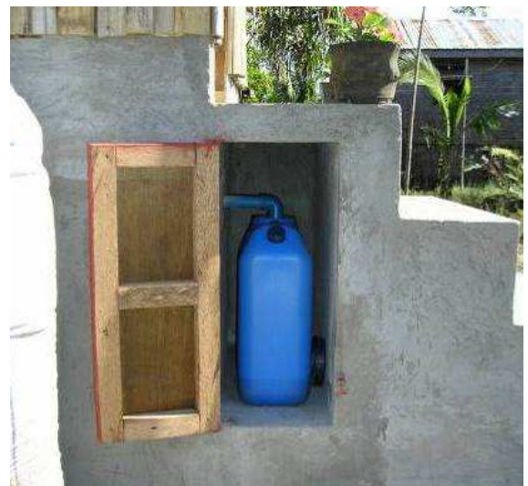
Fig. 9 Urine container, UDDT in barangay Villareal, 2007 (source: DILG-GTZ Water and Sanitation Program)
