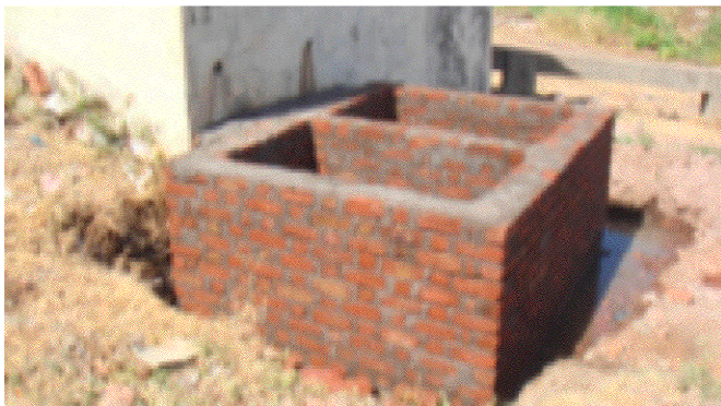
Fig 4: Organic filter for...(under construction) where? Month , year (photo: N. Zimmermann)
