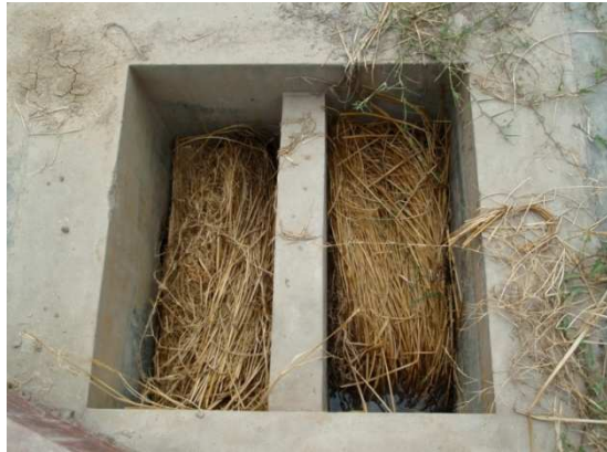
Fig. 12: Organic straw filter at the dishwashing stand (source: secon GmbH, which year?)
