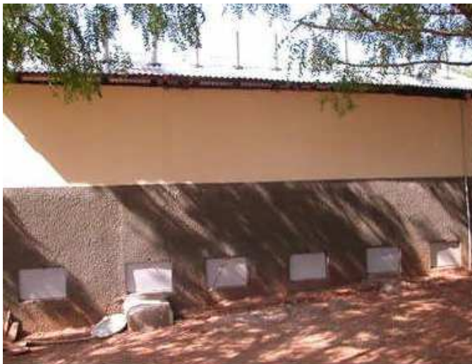
Fig. 6: New "compost" pit latrines for patients, rear view, showing access openings for the removal of faecal sludge (source: EcoSan Club, 2004)
