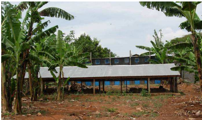
Fig. 9: Covered drying area for collected faeces from UDD toilets (source: EcoSan Club, year?)
