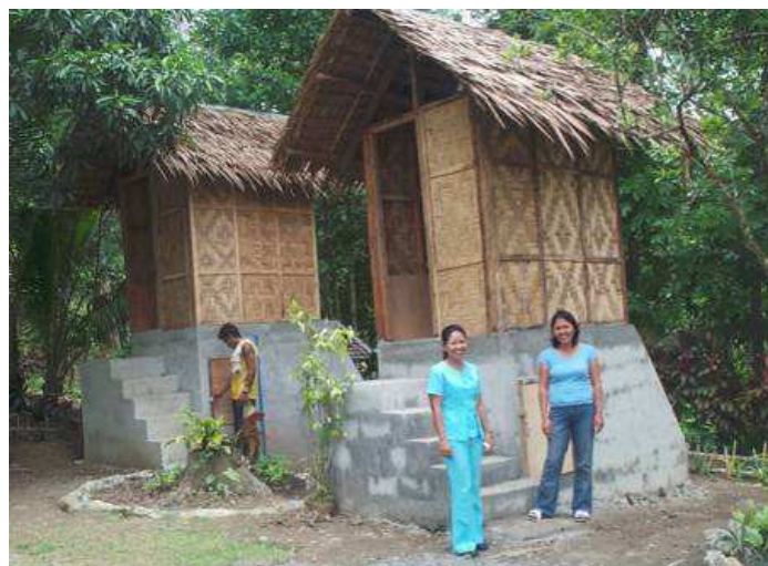
Fig. 4 Two double-vault ecosan UDD toilets in Sinalac Elementary School in Initao Municipality – one for boys, one for girls. The school has 230 pupils; it also has 2 conventional toilets, being pour-flush with pit (photo: E. Sayre, Feb. 2008).
