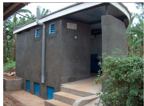
Fig. 6: Demonstration UDD toilet for teachers and visitors (source: EcoSan Club, year?)
