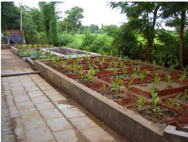
Fig. 9: Elevated (why "elevated"?) gardens for the treatment/reuse of greywater (source: seecon GmbH, which year?)
