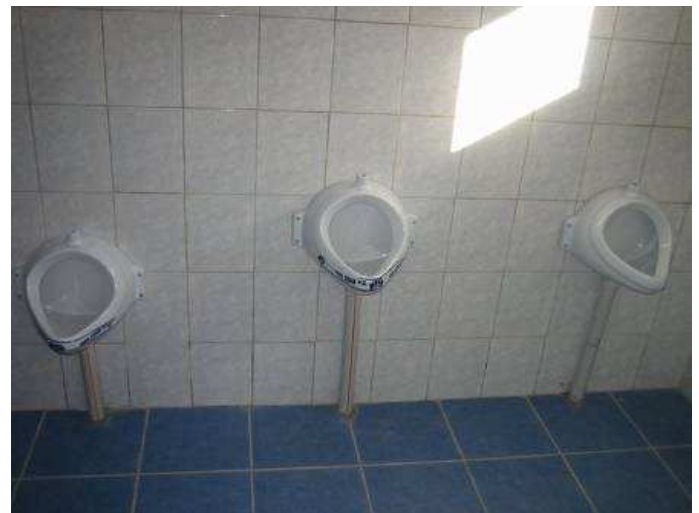
Fig. 10: Boys' waterless urinals at different heights (source: AWHEE, 2006)
