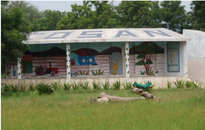
Fig. 5: New sanitation complex with 22 pour-flush toilets and biogas plant (source: seecon GmbH, which year?)
