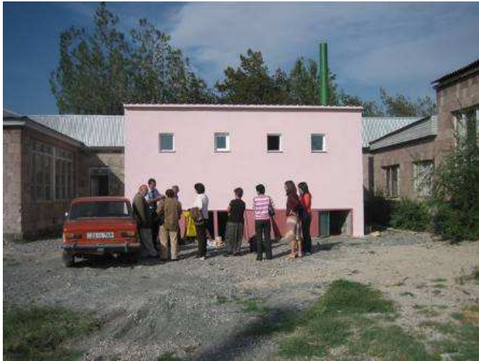
Fig. 5: The new ecosan UDD toilet facility (with 7 cubicles for 350 students) (source: AWHHE, 2006)
