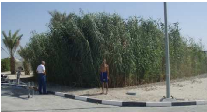
Fig. 10 Reed bed plant for wastewater in Jadaf (source: Waagner Biro Gulf)
