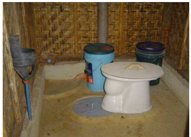
Fig. 8 Inside a UDDT, barangay San Miguel, 2008 (source: DILG-GTZ Program). Note waterless urinal on the left. Area for anal washing in the far left corner.
