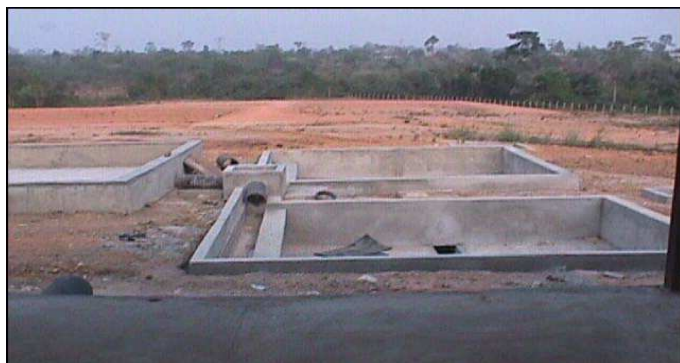
Fig. 4: Faecal sludge drying beds (source: Olufunke Cofie, 2002).
