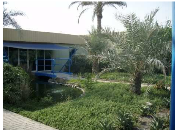
Fig. 9 Greywater garden (source: Waagner Biro Gulf)
