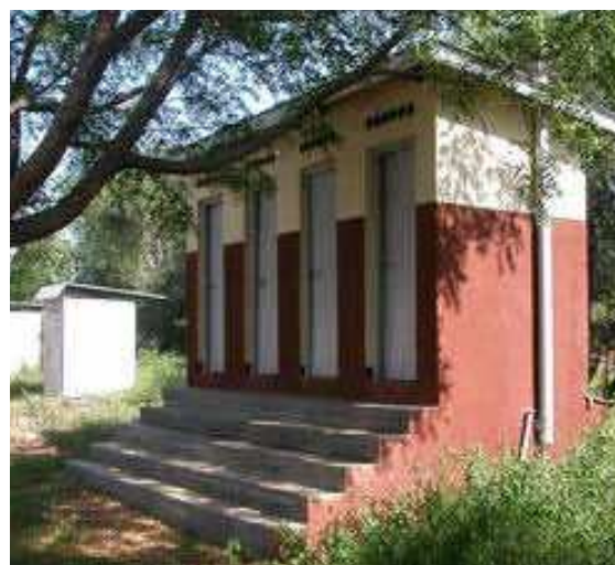
Fig 4: New UDD toilet block with 4 cubicles for the staff (source: EcoSan Club, 2004)
