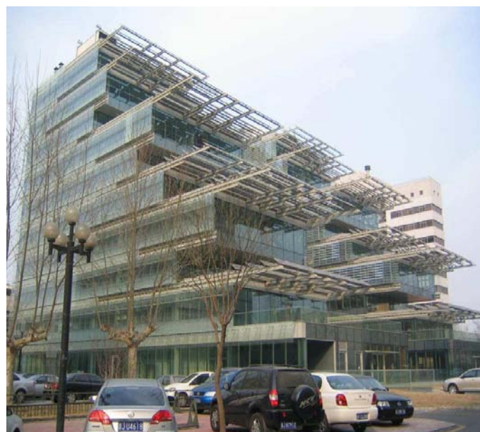
Fig. 3: Sino-Italian Environment & Energy Building at Tsinghua University, Beijing (source: EnviroSystems)
