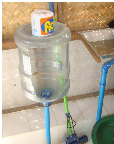
Fig. 7: The recycled water container serves as waterless urinal for men while the sink next to it is for hand-washing. Below the sink is a bucket that contains collected rainwater for handwashing with soap (Source: PUVeP, 2008).
