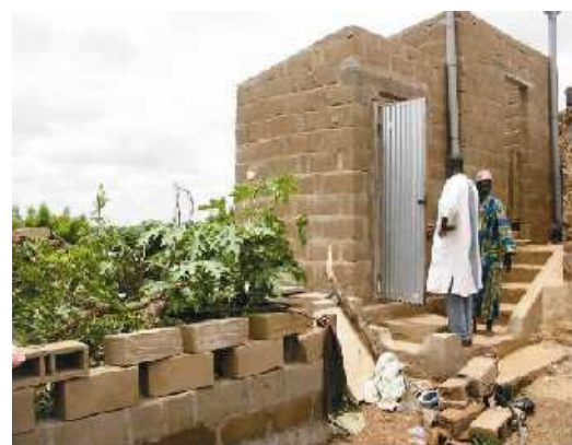
Fig. 3: Ecosan UDD toilet in Koulikoro with shower and greywater garden in 2002 (source: GTZ, 2002).
