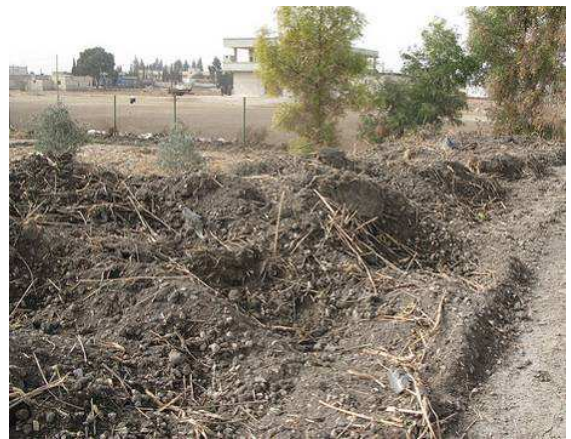
Fig. 11: Mineralised, earth-like sludge taken out of the reed bed used for sludge treatment (after 8 years of operation) – this reed bed used to be where there is now liquid sludge in previous picture (source: E. v. Münch, Jan. 2009).
