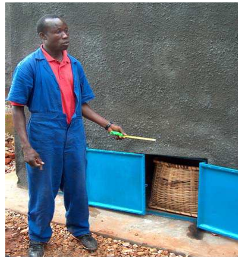
Fig. 7: Wooden faeces collection basket in vault of UDDT (source: EcoSan Club, year?) (who is this person? Maintenance staff?)
