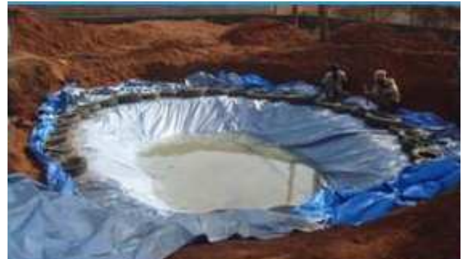
Fig 6: Construction of polishing cum storage pond (photo: N. Zimmermann)
