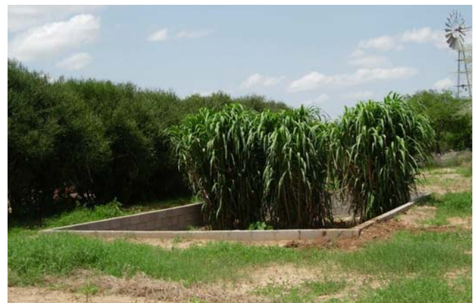
Fig. 8: Constructed wetland in 2006 (source: EcoSan Club)
