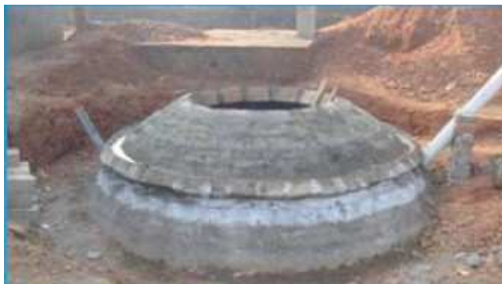
Fig 4: Biogas settler (under construction) (left) and (right) (photo: N. Zimmermann)
