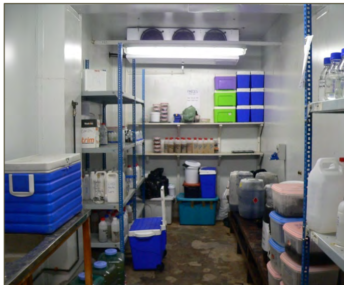
Cold Room – Inside View
