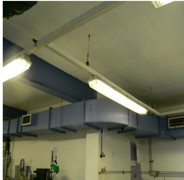
Ventilation System and Air- Conditioning Duct
