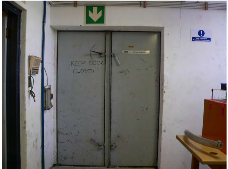
Ground Floor Large Access
