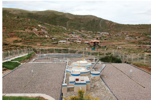
Figure 3. Decentralized wastewater treatment plant at Lomas del Pagador, Bolivia
