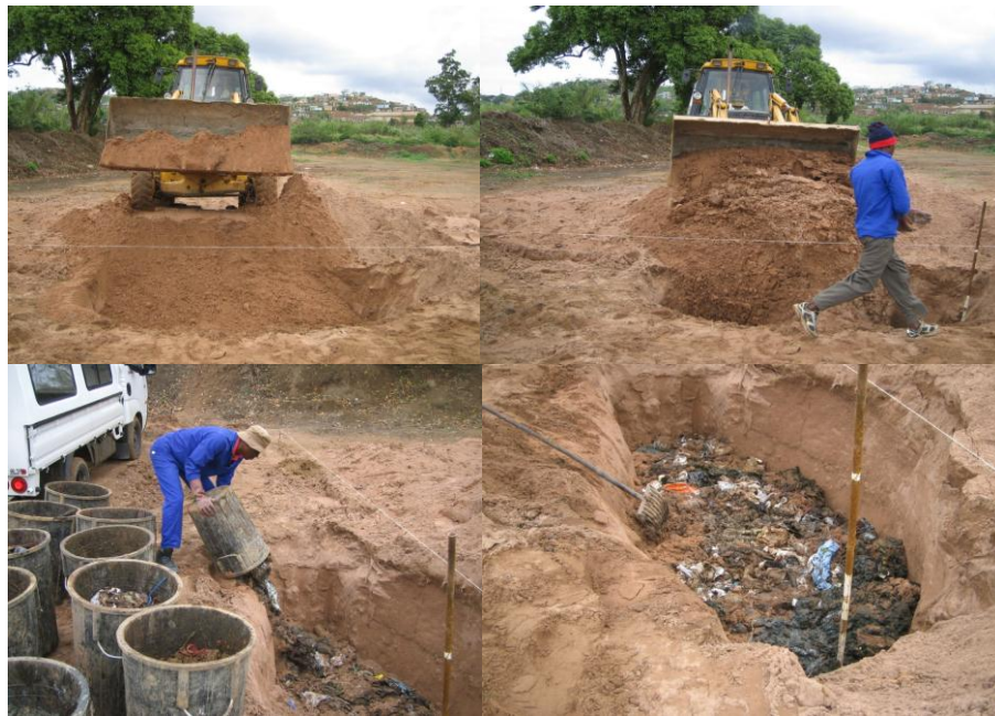
Figure 3.1: Excavation and Sludge burial in Trenches at the Umlazi Site
