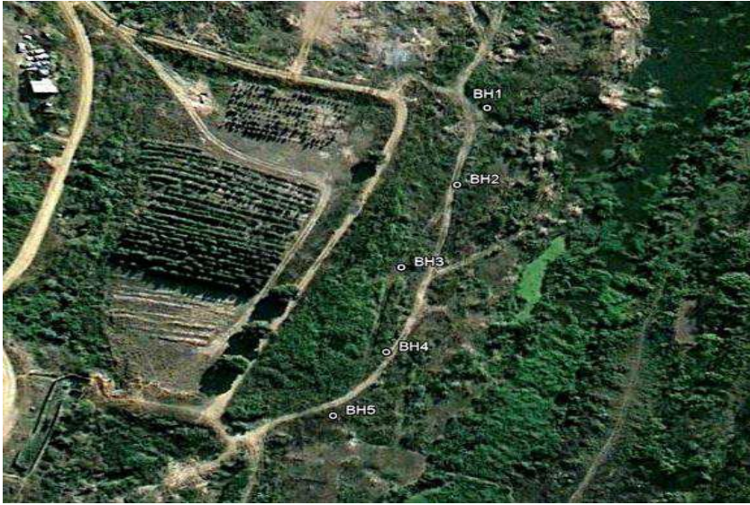
Figure 3.2: Location of boreholes at the umlazi E-pond entrenchment site
