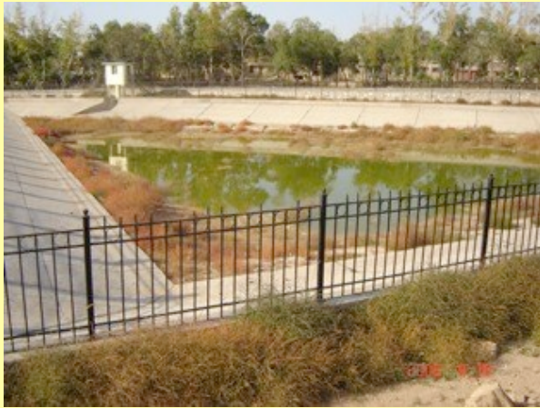
Post-treatment pond (3800 m 3 ) To store the treated GRW and further improve the quality
