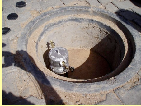
Urine quick coupling in the urine tank
