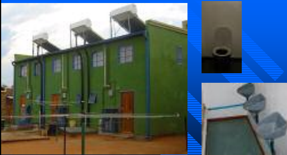
Urine-diverting dry toilets 100 households completed – 2000 planned
