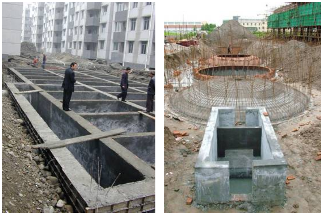
Figure 8: 140.000 Decentralised Wastewater Treatments Systems (DEWATS) have been implemented in China together with the Ministry of Agriculture – many of them in an urban context (Source: Borda).
