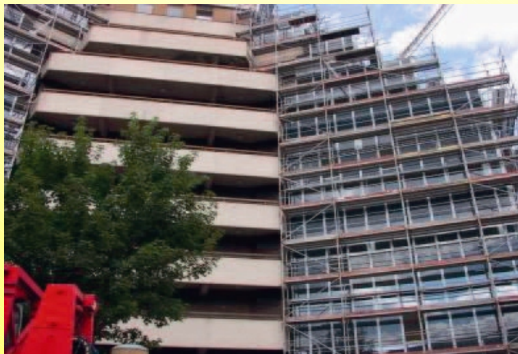
GTZ main office building under construction (GTZ)
