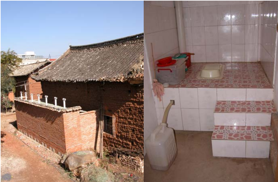
Figure 2: urine-diverting dry toilets (source: Medilanski)
