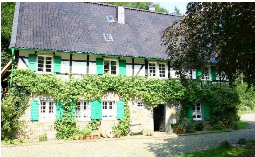
Figure 1: The historical watermill Lambertsmuehle (photo: GTZ)
