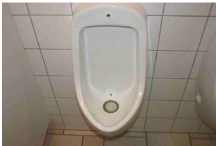
Figure 2: Waterless urinal (photo: Otterwasser)
