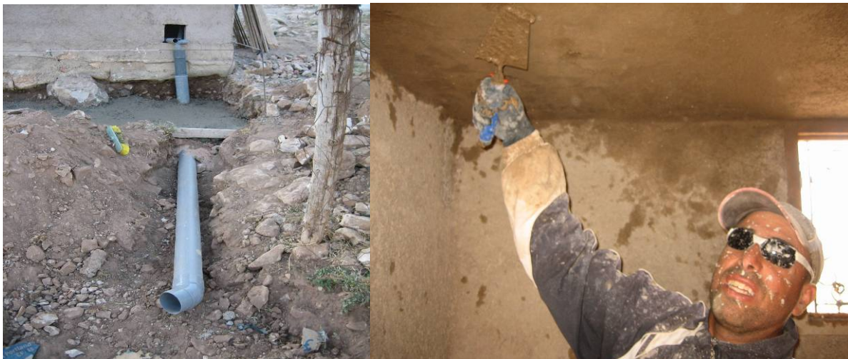
Fig. 68: Installation of urine-pipe (left) and plaster of ceiling (right) at Ferhaoui
