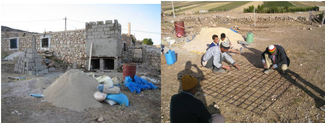
Fig. 63 : Finalise walls (left) and preparing iron for roof-plate (right) at Ahnuch,
