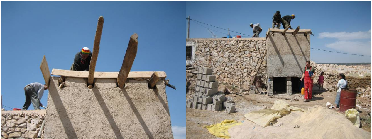
Fig. 73: Formwork for (left) and pouring of roofplate (right) at Ahnuch
