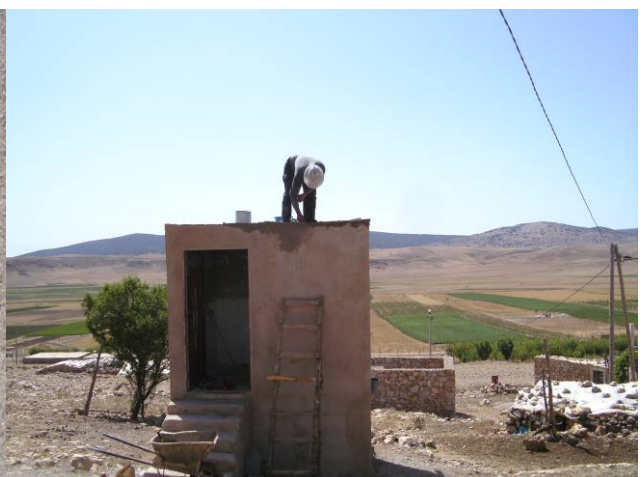
Fig. 81: Plaster of wetland, beigewater-infiltration (left) and sealing of roof (right) at Ferhaoui
