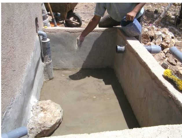
Fig. 87 : Repairing of broken floor of wetland at Ferhaoui, compare Fig. 83
