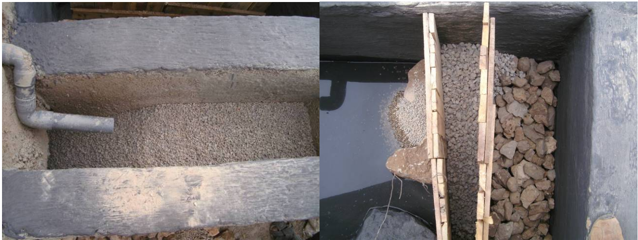
Fig. 101: Beige-water-filter (left) and inflow-area of wetland (right) at Ferhoui
