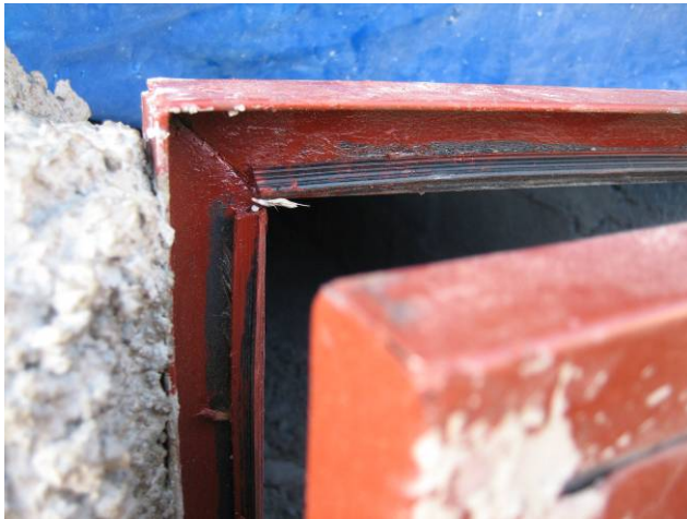
Fig. 5: Sealing of Faeces-chamber-door with rubber
