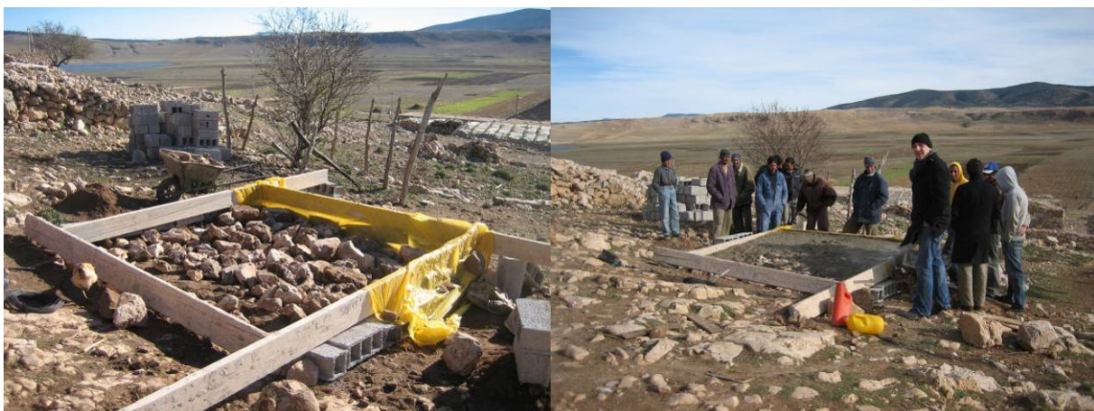
Fig. 21 : Finished formwork for foundation, interested neighbours watch pouring concrete
