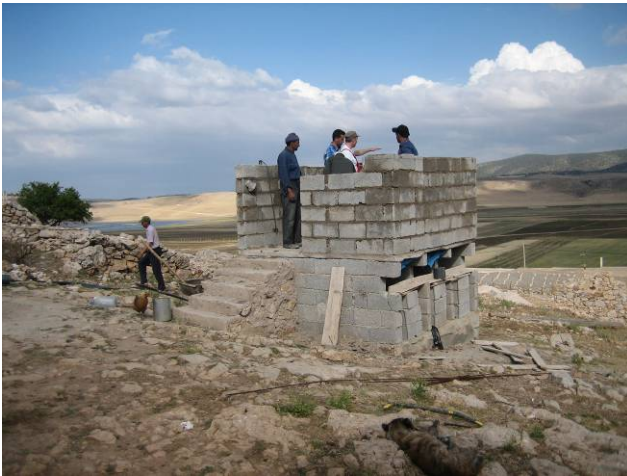
Fig. 41 : Building superstructure-walls at Ferhoui
