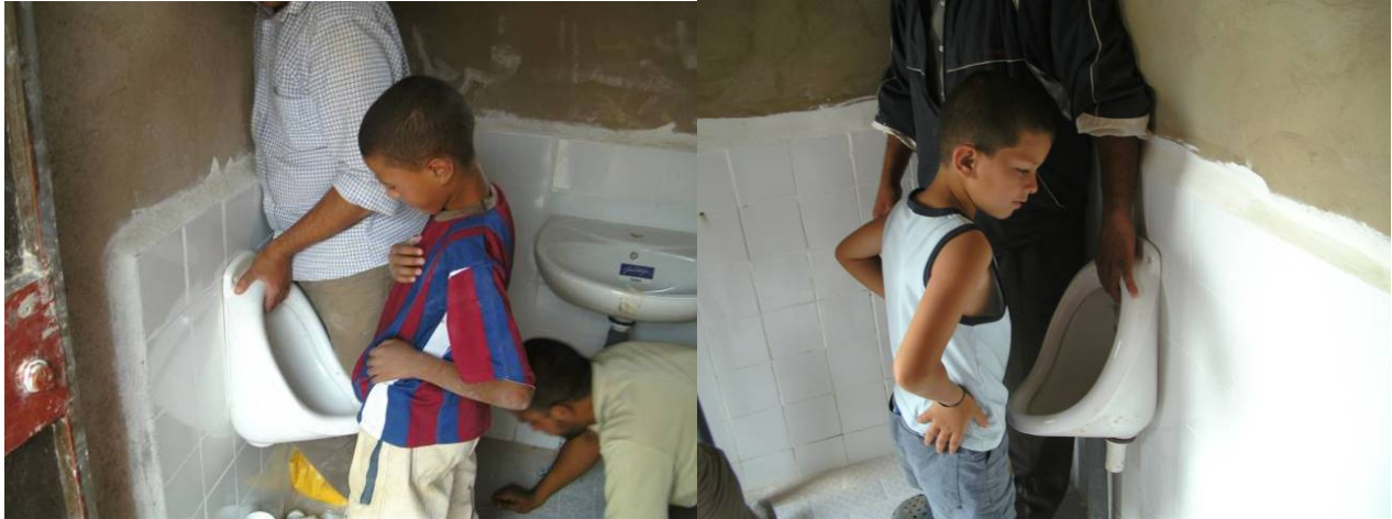
Fig. 96 : Adjusting height of urinal at Jane (left) and Ferhoui (right)
