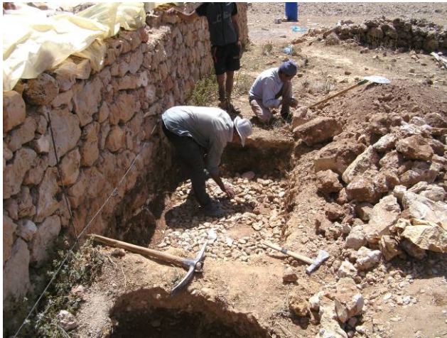
Fig. 82 : Preparation for floorplate of wetland and urine-tank at Ahnuch
