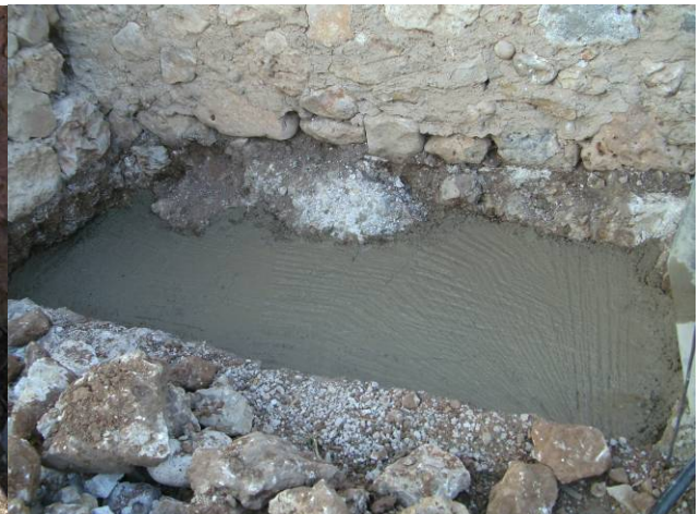
Fig. 66 : Preparation (left) and finished floorplate of wetland at Khaled
