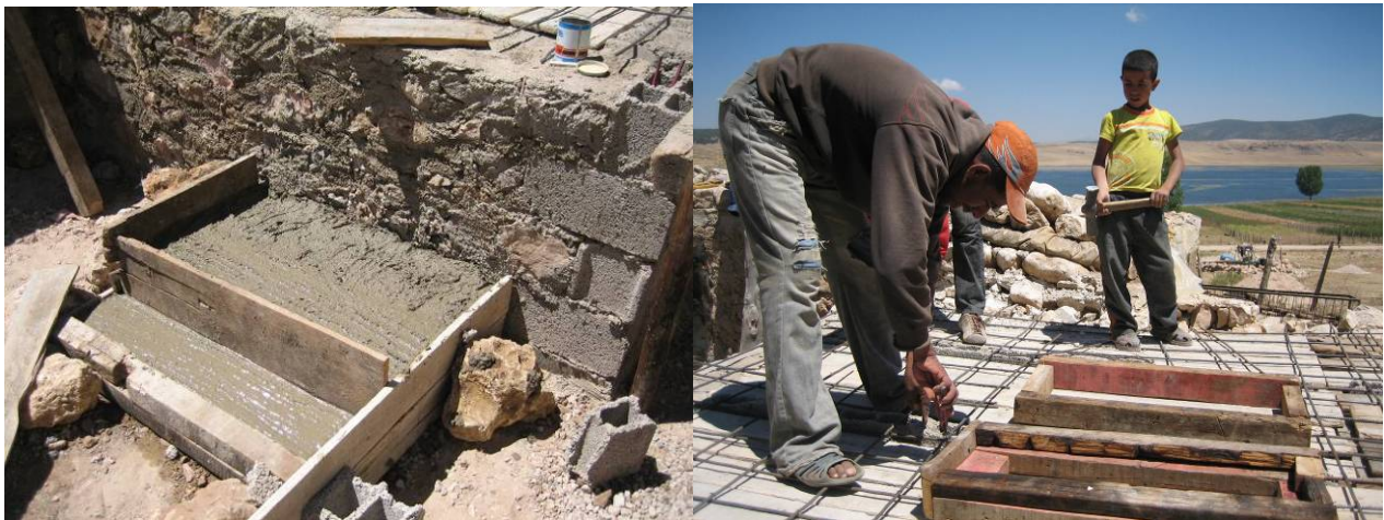
Fig. 47: Building stairs (left) and preparation for plate at Khaled (right)
