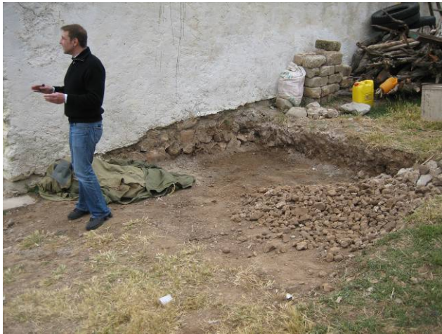
Fig. 32 : Place for Toilet of Fam. Jane, Excavation work already started
