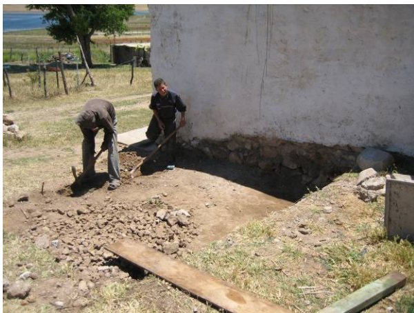
Fig. 35 : Foundation works Fam. Jane
