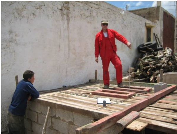
Fig. 43: Building the formwork and iron for the plate
