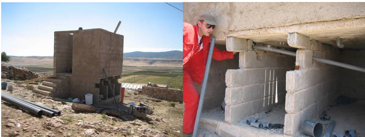
Fig. 51 : First layer of plaster (left) and start sanitary installations at Ferhoui
