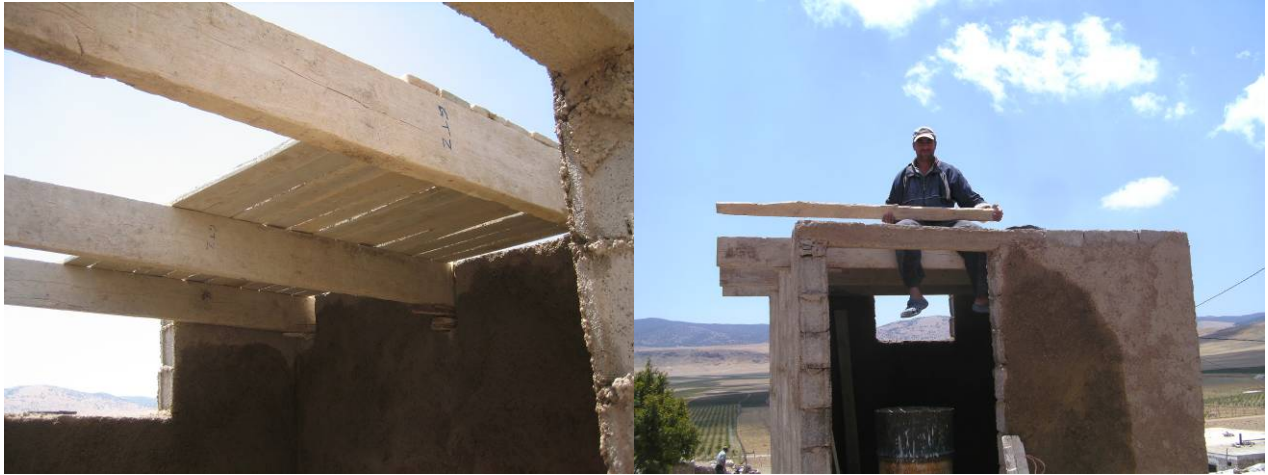
Fig. 52 : Formwork for roofplate at Ferhoui
