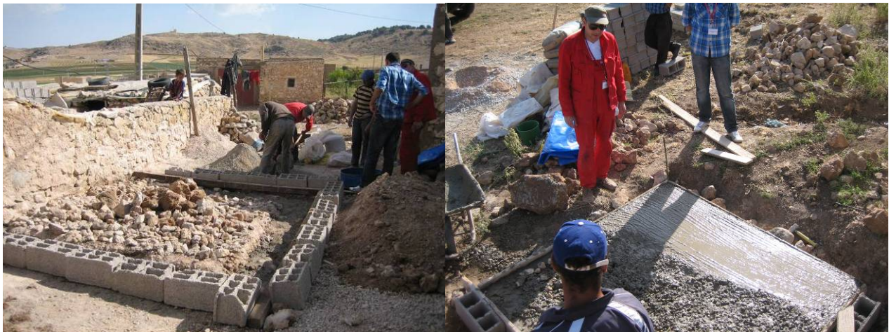
Fig. 39 : Pouring foundation at Fam. Khaled (left) and Ahnouch (right)
