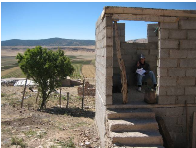
Fig. 44 : Building beam above door at Ferhoui
