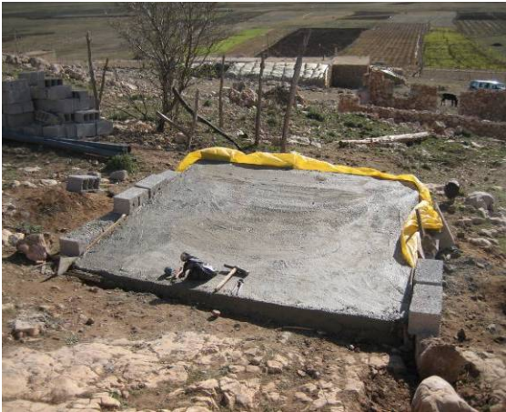
Fig. 22: Finished foundation
