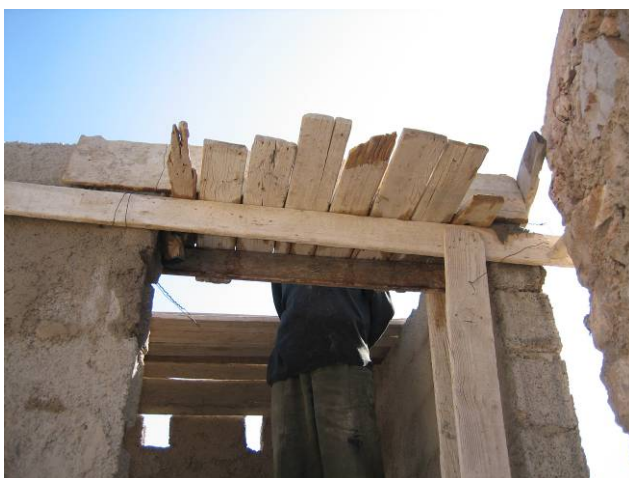
Fig. 69: Formwork for beam above door at Ahnuch
