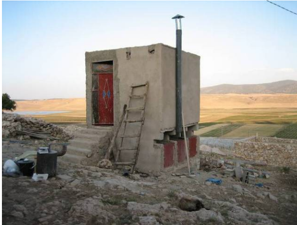
Fig. 64 : Ferhaoui-UDDT almost finished
