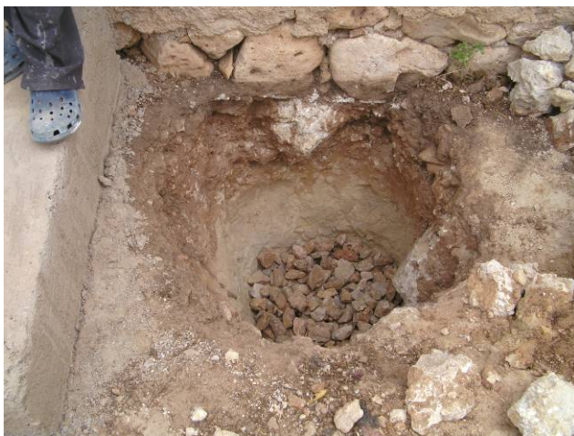
Fig. 100 : Infiltration-drainage-layer at Khaled
