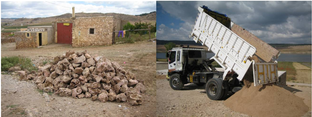
Fig. 34 : Natural stones for Construction of UDDT for Fam. Khaled, sand-delivery
