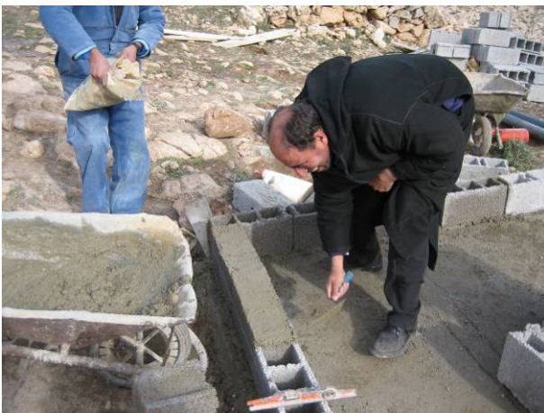
Fig. 23 : Mason building faeces chamber walls
