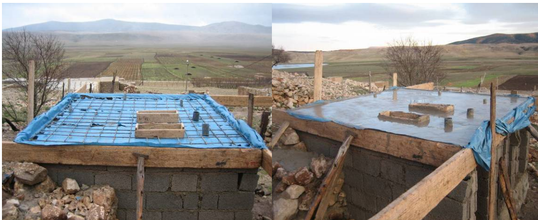
Fig. 29 : Prepared formwork for ground plate and finished ground plate
