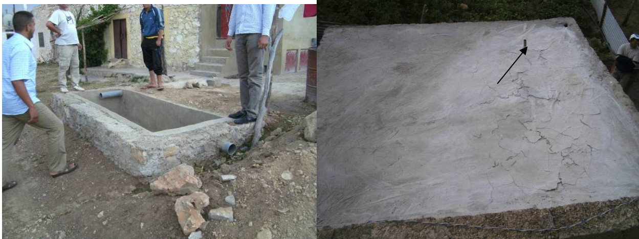
Fig. 75 : Wetland (left) and roof (right) of Jane, note pipe for water-connection !
