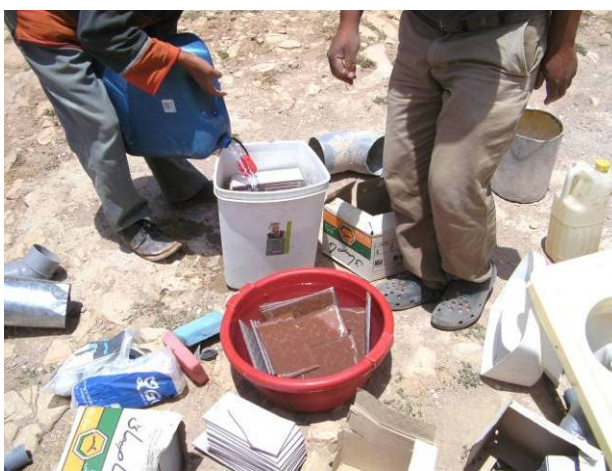
Fig. 92 : Preparing tiles and almost finished floor at Ferhaoui
