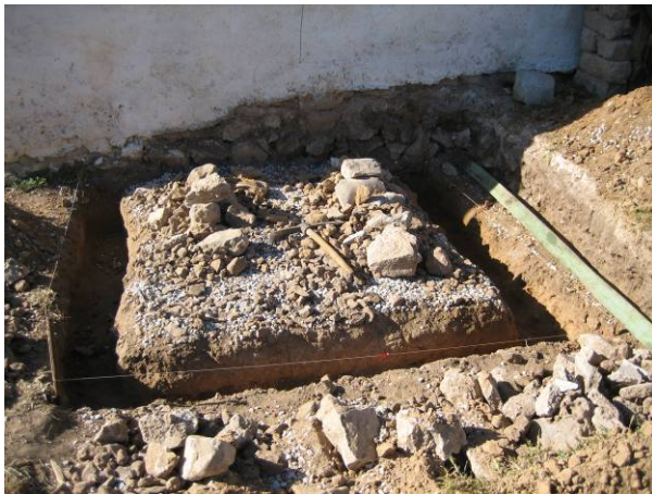
Fig. 4 : Excavation for Round Foundation
