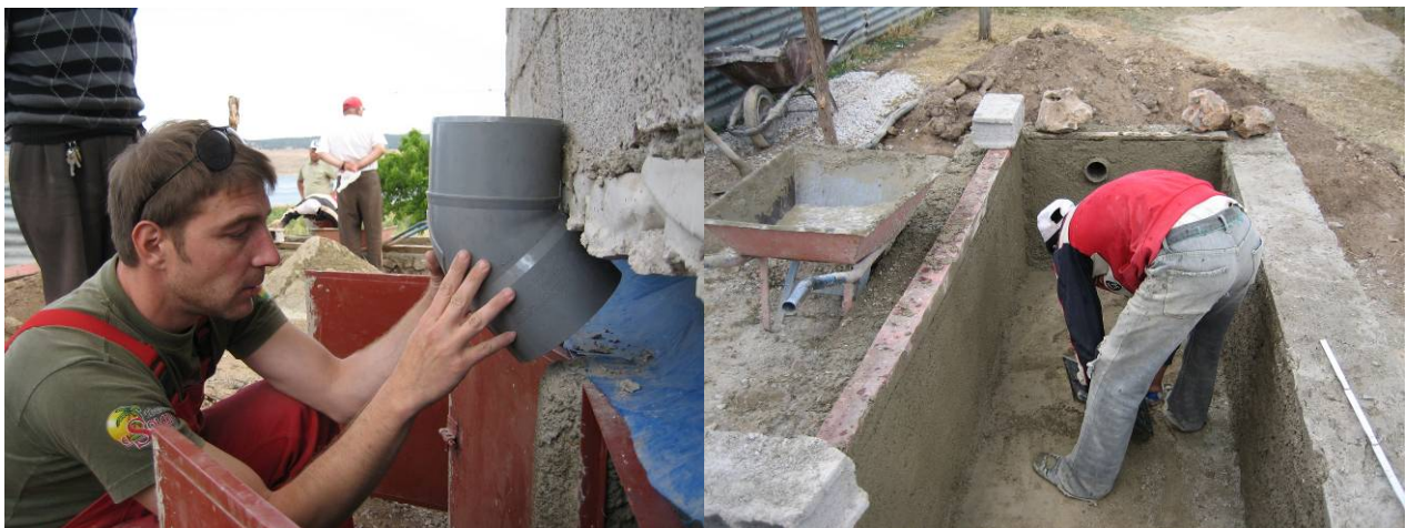
Fig. 71 : Installing ventilation-pipe (left) and plaster of the wetland (right) at Jane
