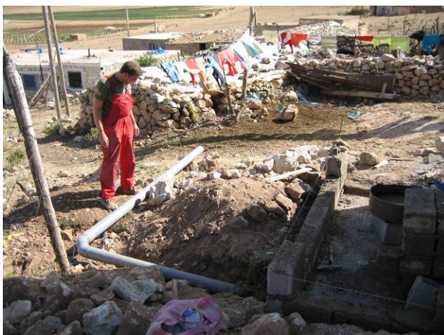
Fig. 72 : Building walls of wetland and urine-pipeline at Ferhoui
