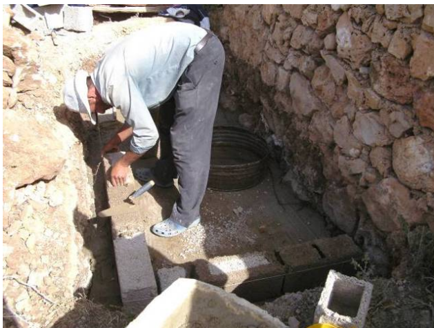
Fig. 86 : Building walls of wetland at Ahnuch
