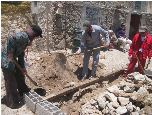
Fig. 38 : Preparation of formwork for foundation at Khaled
