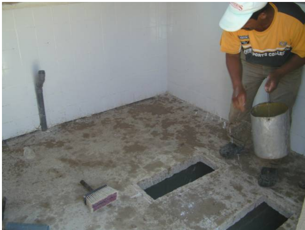
Fig. 91 : Preparing floor for tiles at Jane
