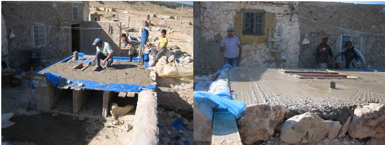
Fig. 49: Pouring (left) and finalised plate at Khaled
