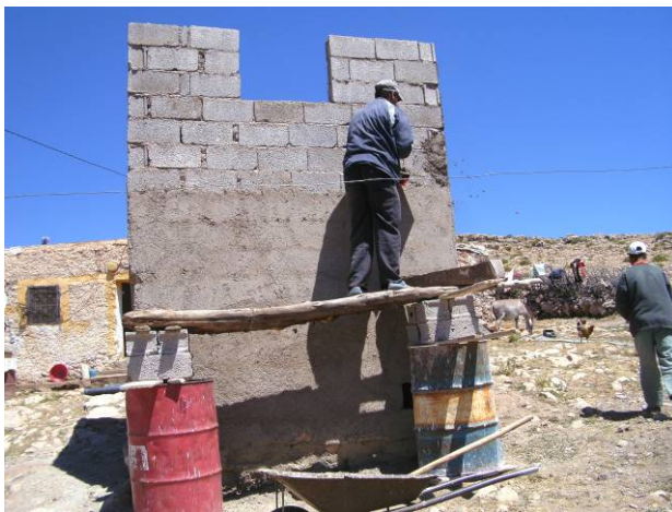
Fig. 48: Plastering of the walls at Ferhaoui
