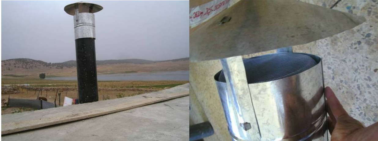
Fig. 10 : rain-cap of vent-pipe with flynet
