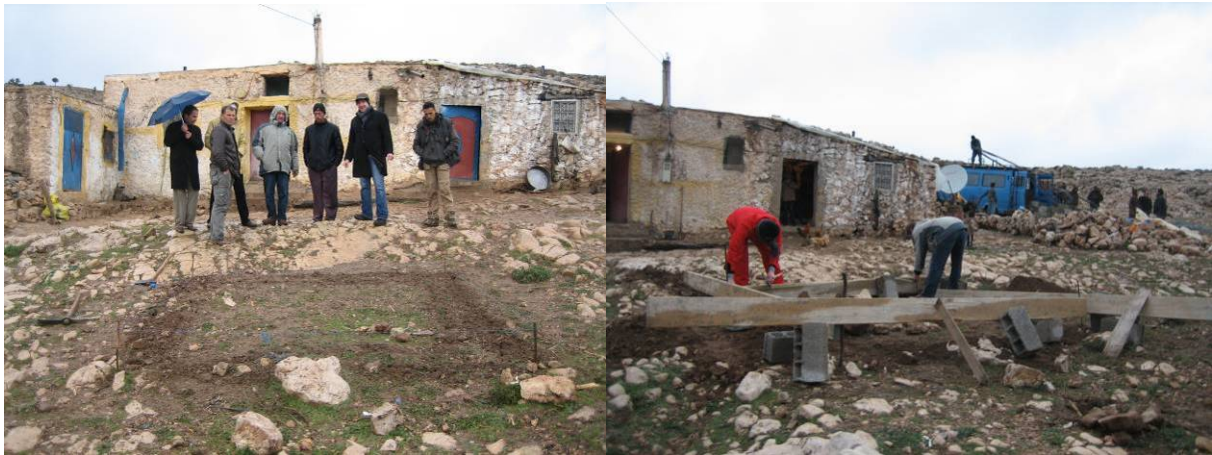
Fig. 20 : Place and setting the formwork for foundation at Ferhoui
