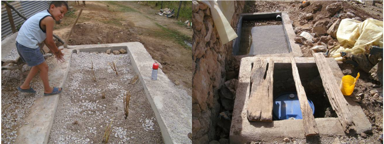
Fig. 99 : Planting reed at Jane (left) and urine tank/ constructed wetland at Ahnuch (right)
