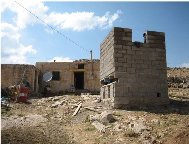
Fig. 42 : Almost finished walls at Ferhoui
