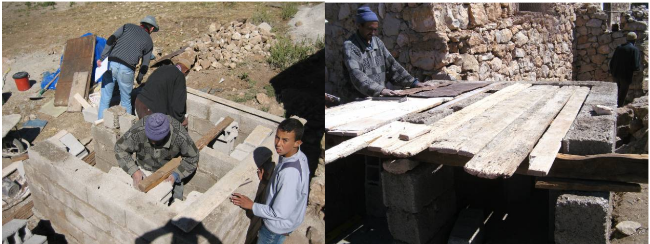
Fig. 45 : Support for and lower formwork for plate at Ahnouch
