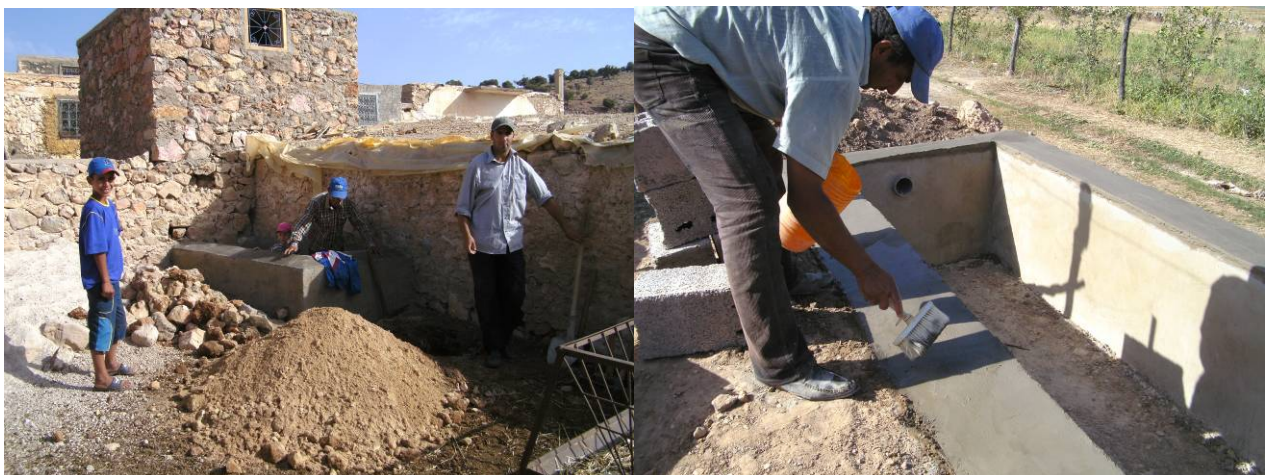
Fig. 84 : Plaster of wetland at Khaled (left) and Jane (right)
