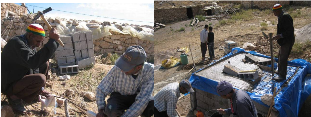
Fig. 50 : Cutting iron for plate and pouring plate at Ahnuch
