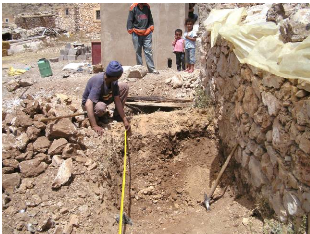
Fig. 78 : Preparation for wetland (front) and urine-tank (back) of Ahnuch
