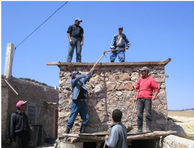
Fig. 65: Pouring roof plate at Khaled
