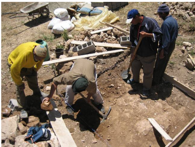
Fig. 37 : Excavation for UDDT at Ahnuch, note rocky ground !
