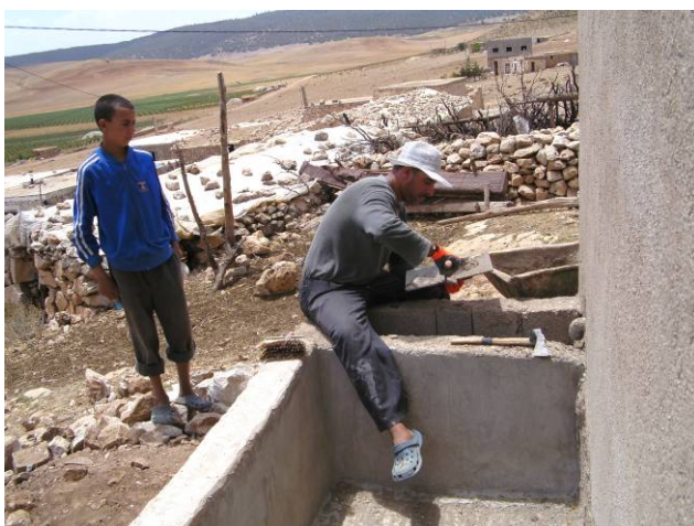
Fig. 81: Plaster of wetland, beigewater-infiltration (left) and sealing of roof (right) at Ferhaoui
