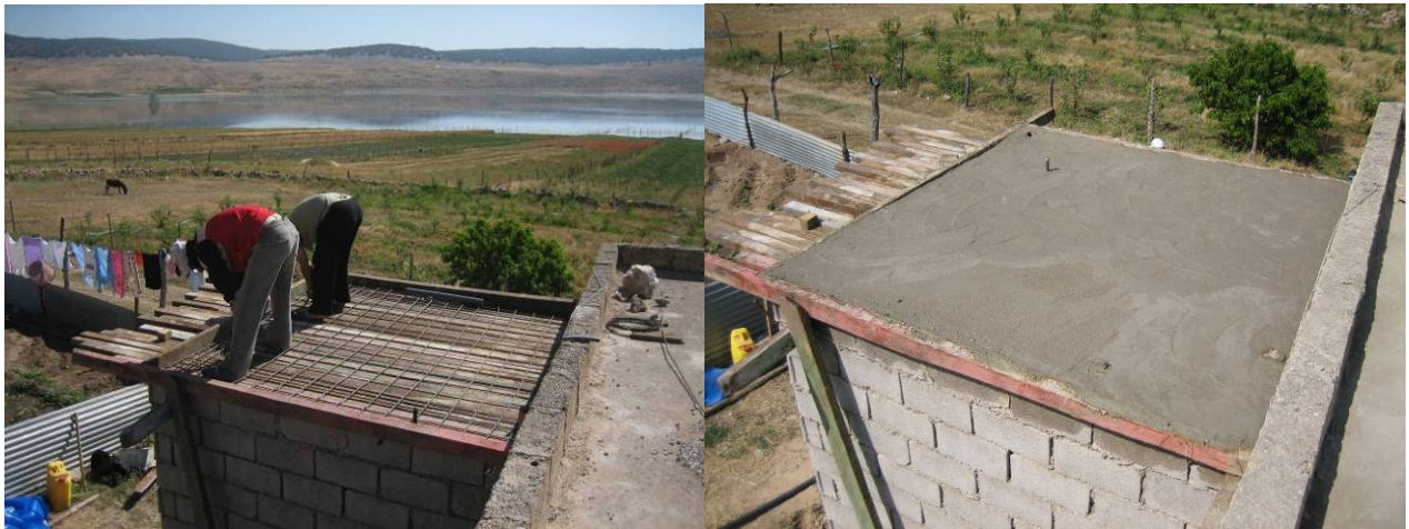
Fig. 56: Formwork and iron for roofplate (left) and finished roofplate at Jane
