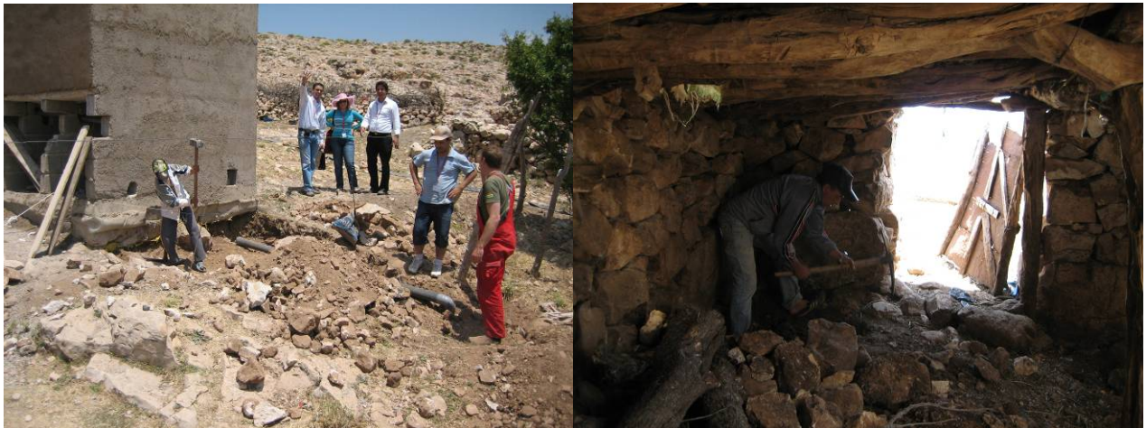
Fig. 57 : Excavation for wetland (left) and urinetank in stable (right) at Ferhaoui,
