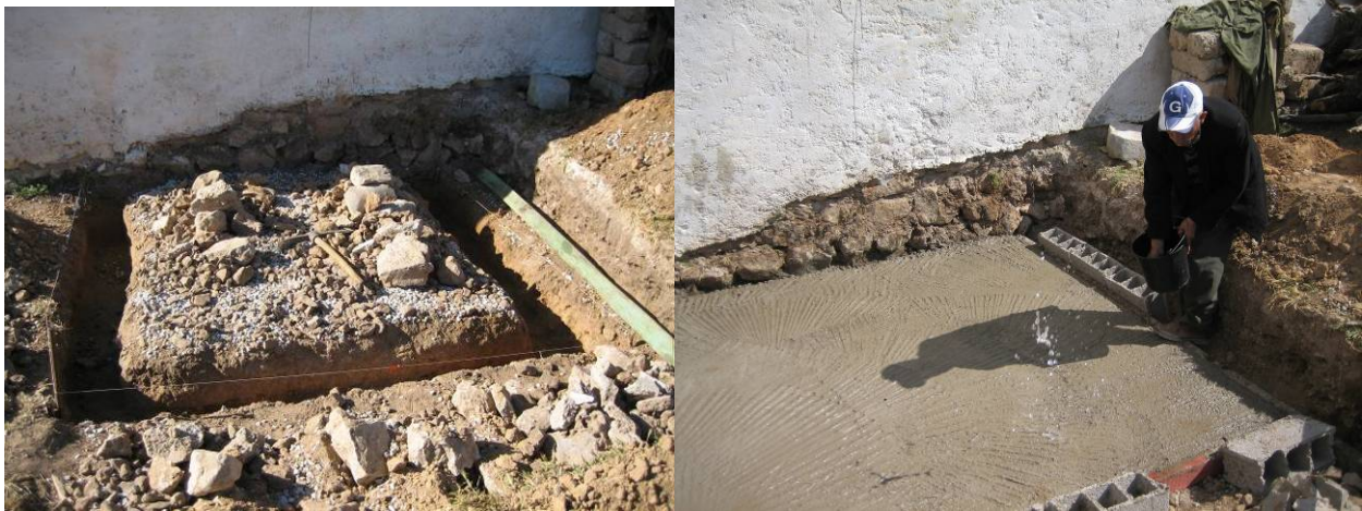
Fig. 36 : Excavation Fam. Jane (left), adding water to finished groundplate (right)
