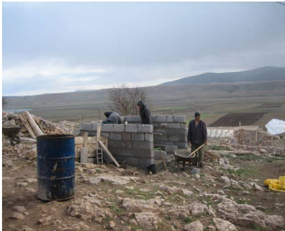
Fig. 27 : Faeces chamber walls and stairs
