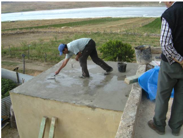
Fig. 80 : Repairing of broken roof at Jane
