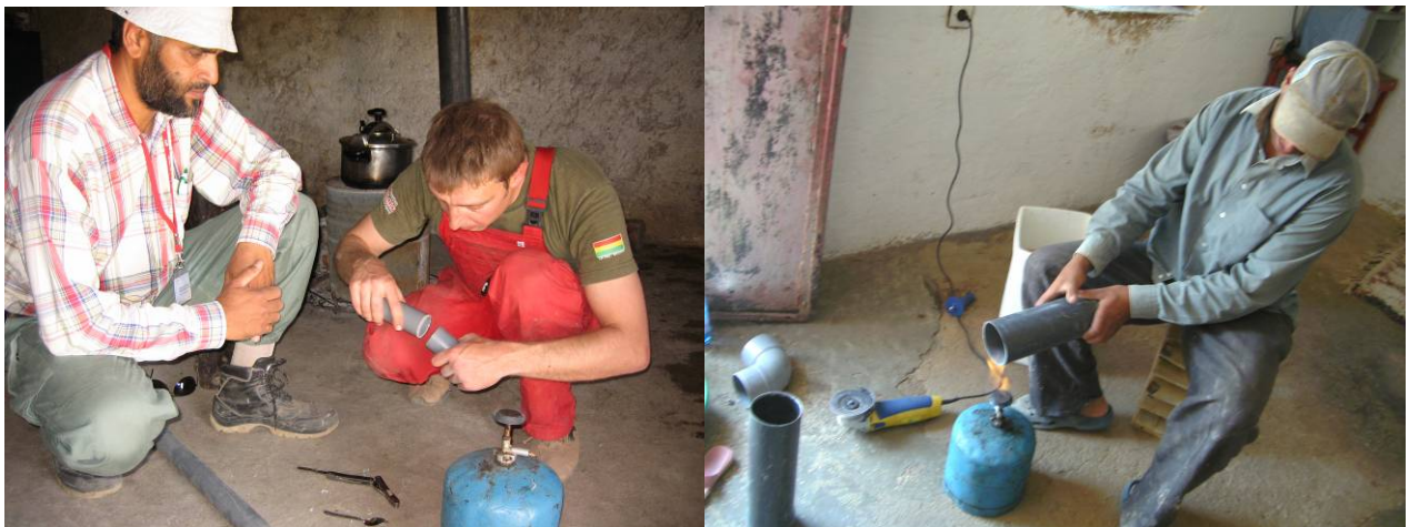
Fig. 58 : Demonstration how to make adapters from PVC-pipes with heat
