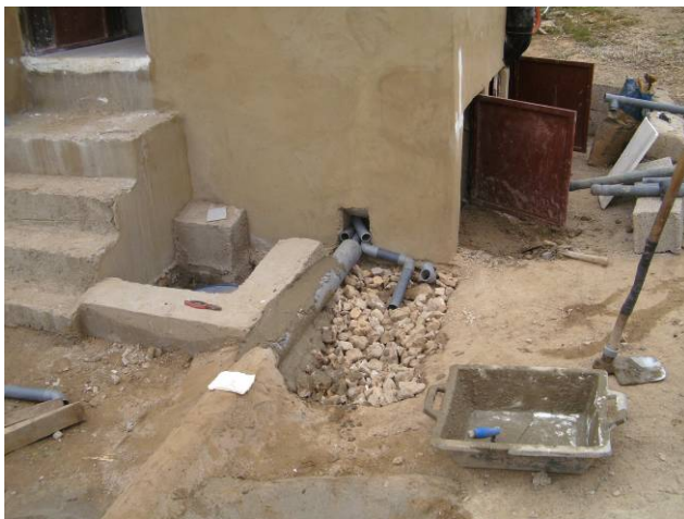
Fig. 97: Urine-Tank (left) and beigewater infiltration (right) at Jane
