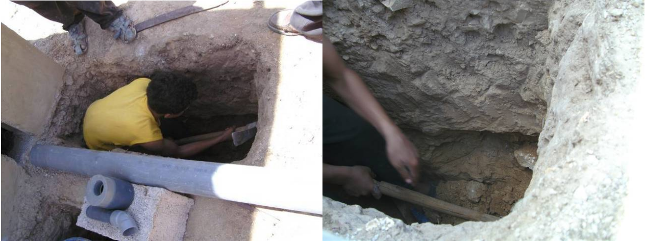
Fig. 88 : Increasing infiltration-area at Jane
