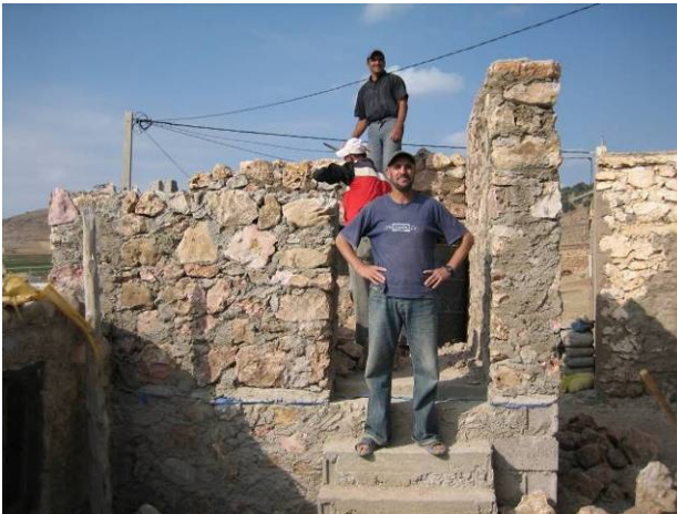
Fig. 60 : Building walls (left) and at Khaled
