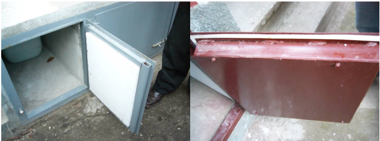
Fig. 6 : Insulation of faeces-chamber-door with styrofoam
