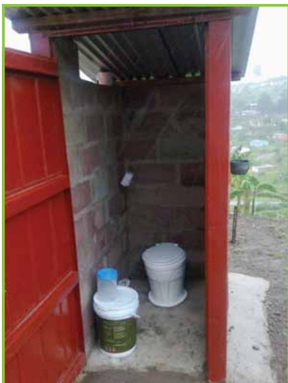
Pour flush toilets selected for conversion to low flush systems
