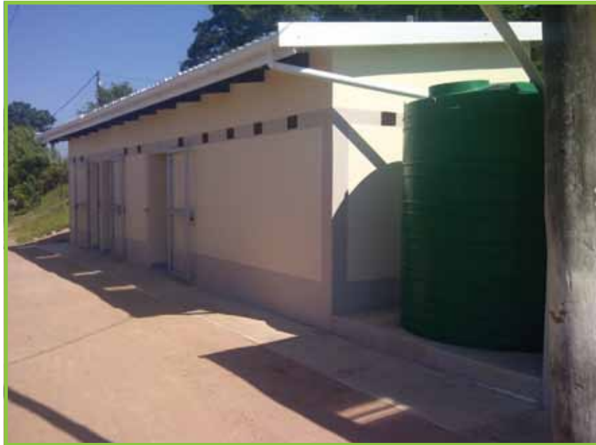
Newly built toilet blocks at Sizimesele Primary School
