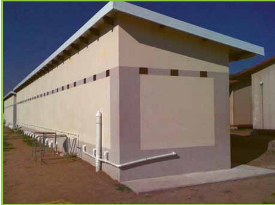
New Toilet blocks at Thandaza High School
