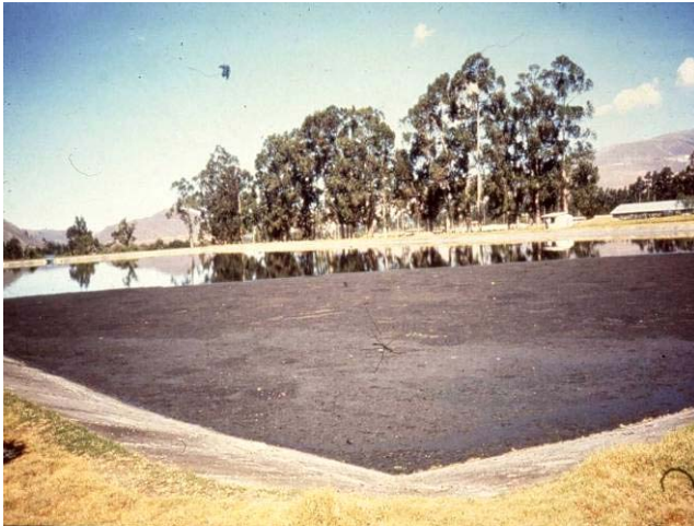
Figure 12. A facultative pond with a high accumulation of scum.
