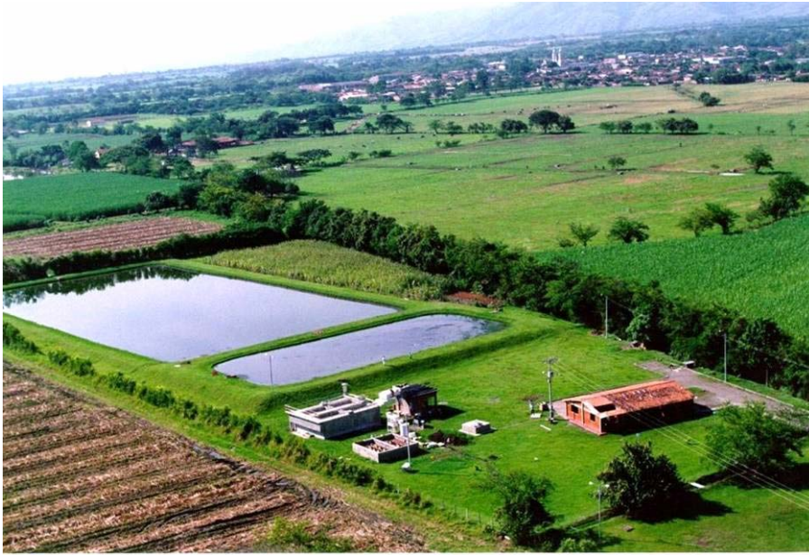
Figure 2. WSP system at Ginebra in southwest Colombia (population 9,000; wastewater flow 27 l/s) comprising an anaerobic pond and a facultative pond. The WSP effluent is used for the irrigation of sugar cane.
