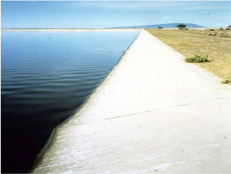
Figure 6. Embankment protection with in situ concrete slabs.
