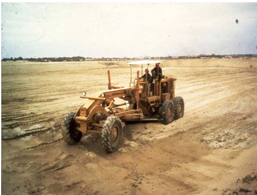
Figure 5. WSP construction – earthmoving is the main activity.
