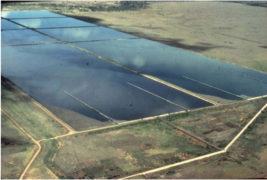
Figure 4. Phase I of the WSP system at Dandora serving Nairobi, Kenya (design flow 30,000 m 3 /d) comprising two series with a facultative and three maturation ponds. [Phase II comprises a further six series to the right of the Phase I series (design flow 80,000 m 3 /d), and Phase III will add an anaerobic pond as the first stage in the eight series (design flow about 160,000 m 3 /d).]
