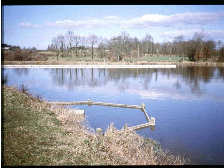
Figure 8. Pond inlet with scum box.
