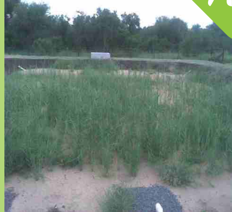
A reed bed under construction - new reeds are planted
