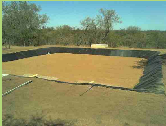
A reed bed under construction: PVC lining and sand
