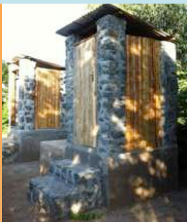
Foreground: Worm toilet Background: Terra Preta Toilet photo taken at Crown Ministries, Malawi
