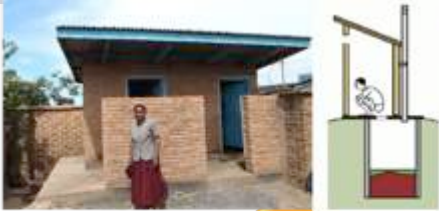
Bangwe Market Pit Latrine Users per day: 50-100 people Sludge age: 2weeks - 1month
