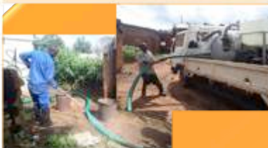
Pit Latrine Emptying High Pressure Fluidisation Vacuum pump
