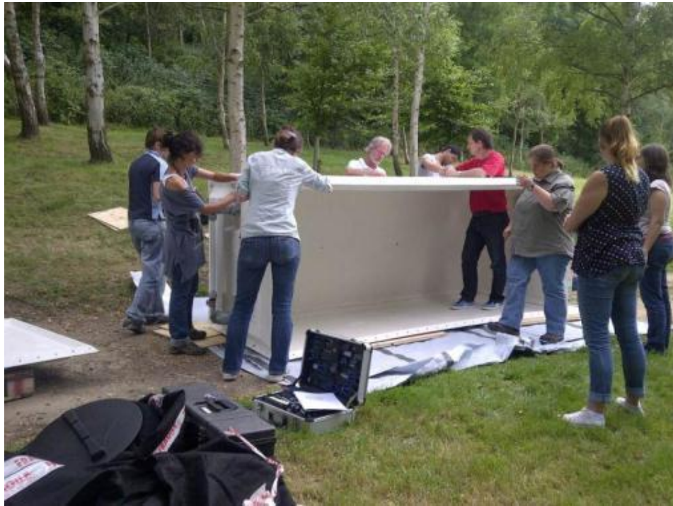
British Red Cross Sanitation Personnel assembling GRP tank
