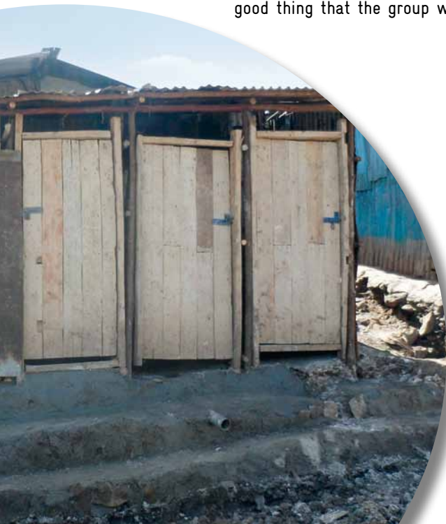
Public sanitation facilities in Mathare
