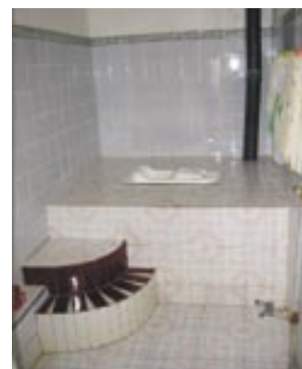
Urine-diverting double-vault dry toilet built indoors (Guangxi Province, China)
