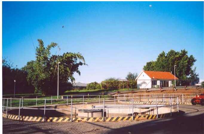
Abbildung 16: Gammams Wastewater Treatment Plant
