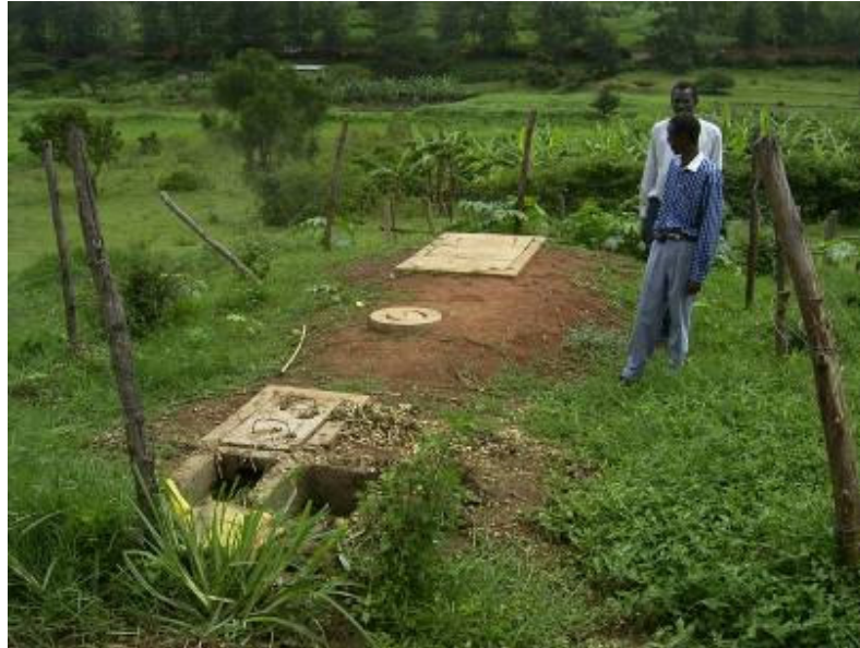
Picture 2: a biogas plant constructed with Chinese assistance. A 3-chamber inlet reduces the risk of short chopped fodder, which is spoiled in the dung, from entering the digester. This reduces the risk of scum formation.
