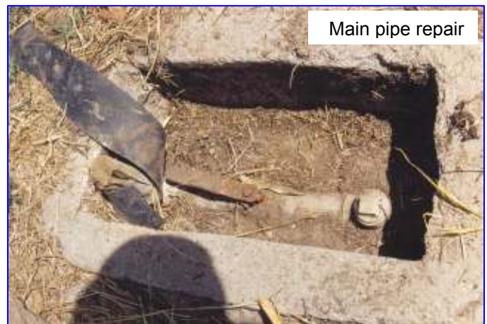
Unblocking inlet pipe
