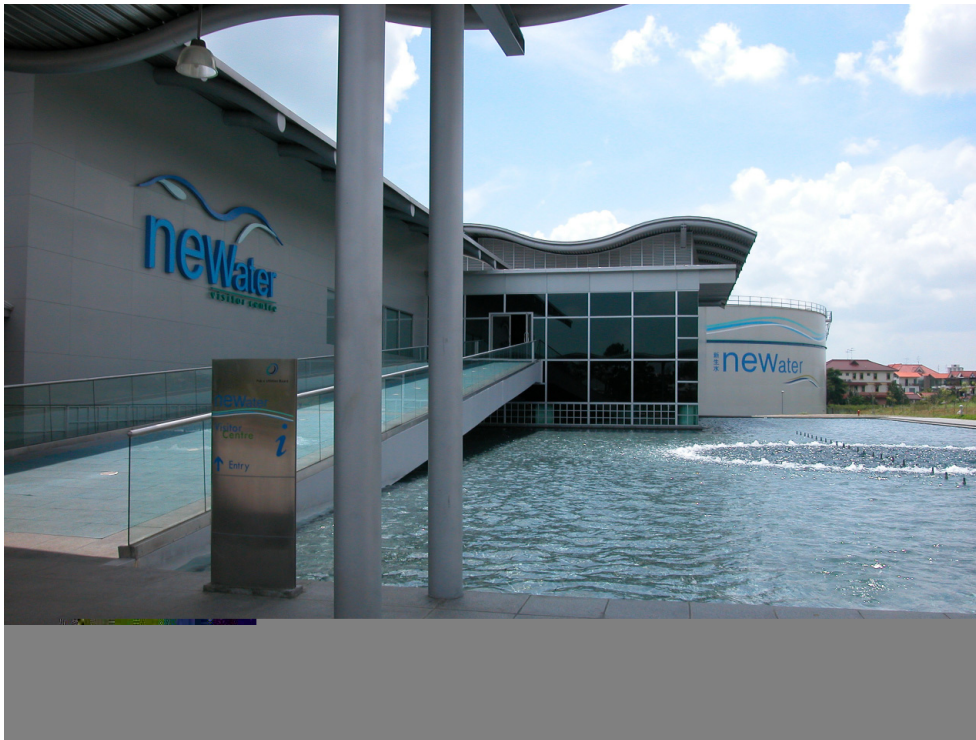
Figure 9.21: NEWater Visitor's Centre in Singapore (Public Utility Board Singapore)
