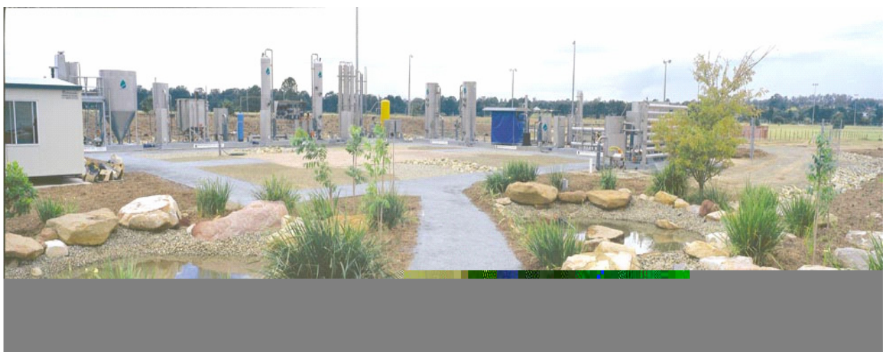
Figure 9.20: Advanced Water Recycling Demonstration Plant in Queensland/Australia (Queensland Environment Agency)
