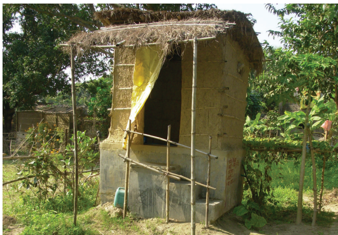
Raised, waterproofed substructures were built with project support (top). Households added their own superstructures (bottom).
