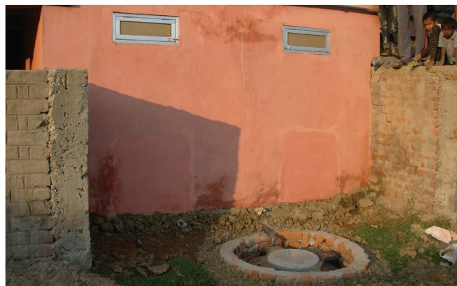
A collection tank for the liquid fertilizer known locally as “fertila” (treated urine and washing water) outside the processing chamber of the sanitation and hygiene complex
