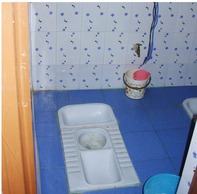
Toilet with squatting pan that separates urine and anal-cleansing water. A rope hanging from the ceiling helps less-able users.
