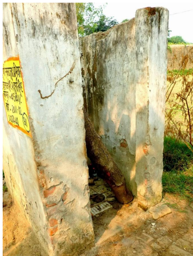
a government-constructed latrine, now out of use
