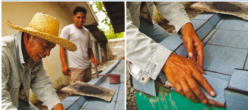
>> Local community members help to construct washing facilities.
