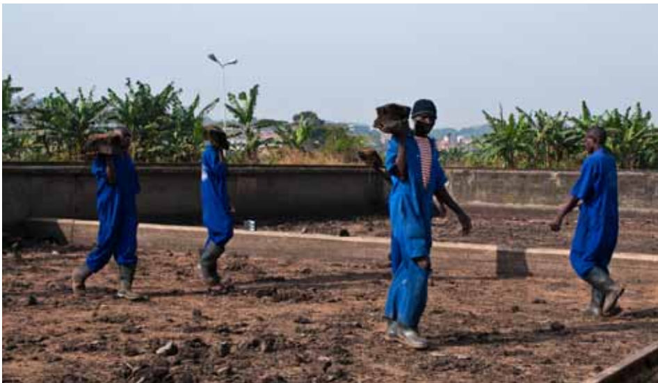
Figure 11.7 Sludge removal from drying beds at the Bugolobi Treatment Plant in Kampala, Uganda (photo: Linda Strande).
