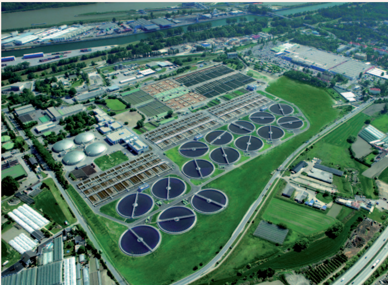
Figure 1: The Vienna main wastewater treatment plant ( http://www.ebswien.at/hauptklaeranlage/service/presse/ )
