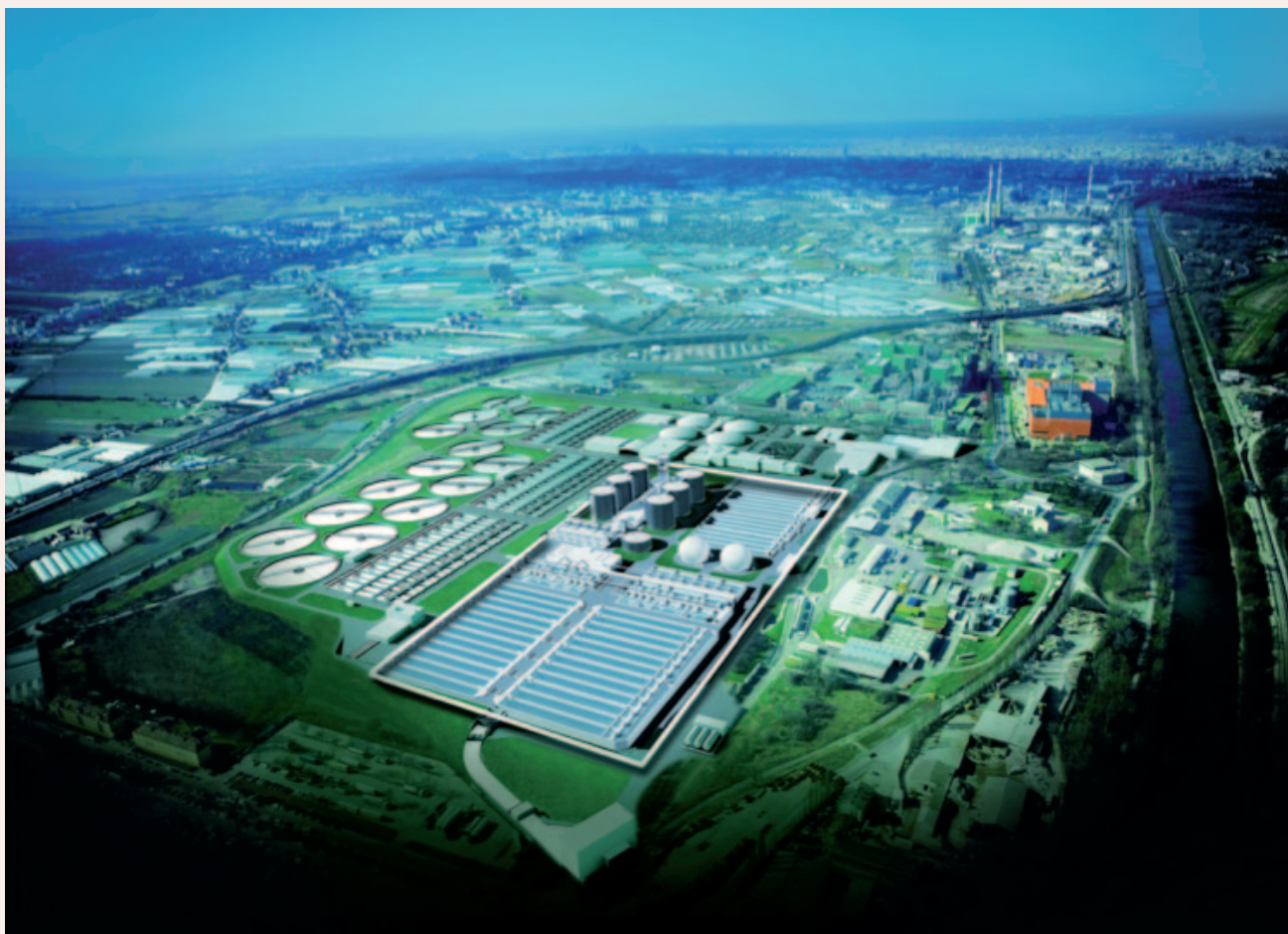
Figure 2: The Vienna main wastewater treatment plant in 2020 (ebs, 2014).
