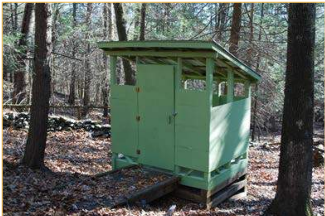
Moldering Privy with Accessible Ramp- A.T. Connecticut
