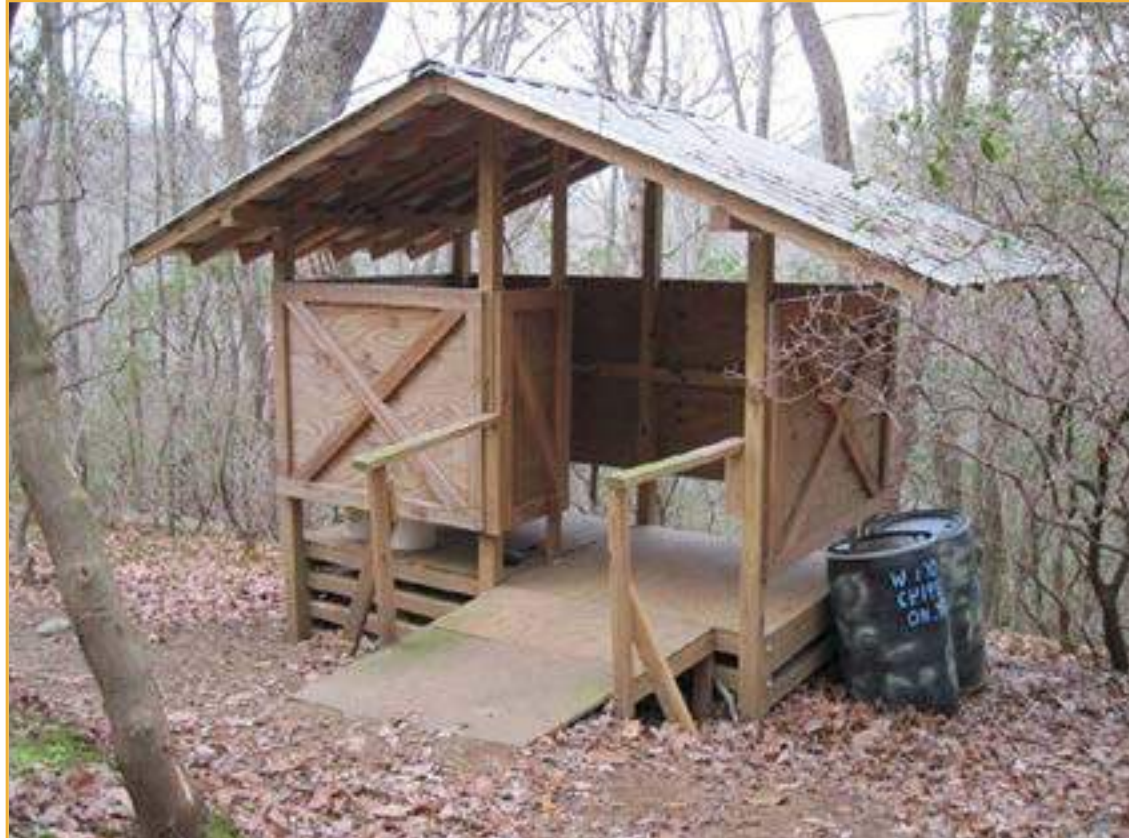
Accessible Moldering Privy
