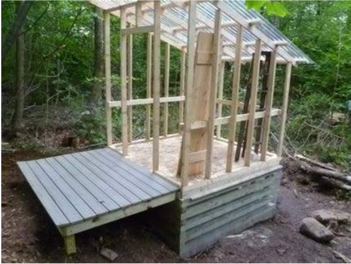
Roof and deck added.
