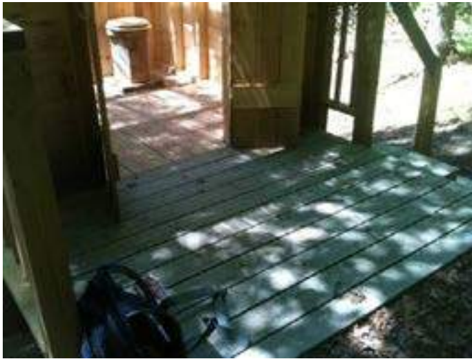
Key Accessibility requirement - the 5'x5' transfer platform
