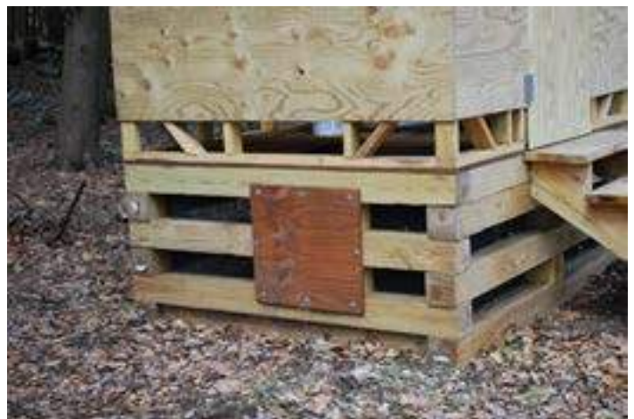
Moldering Privy Crib Access
