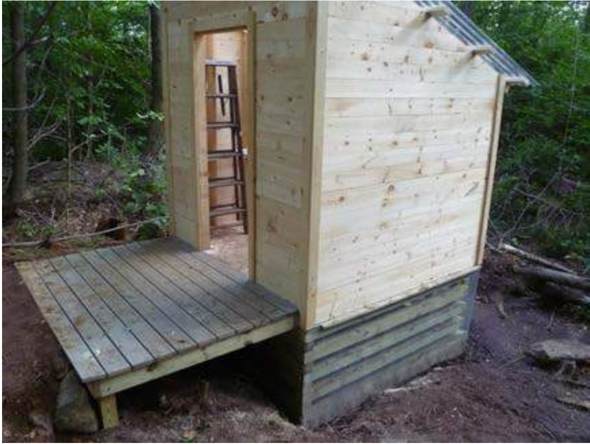
Siding and earth ramp added.
