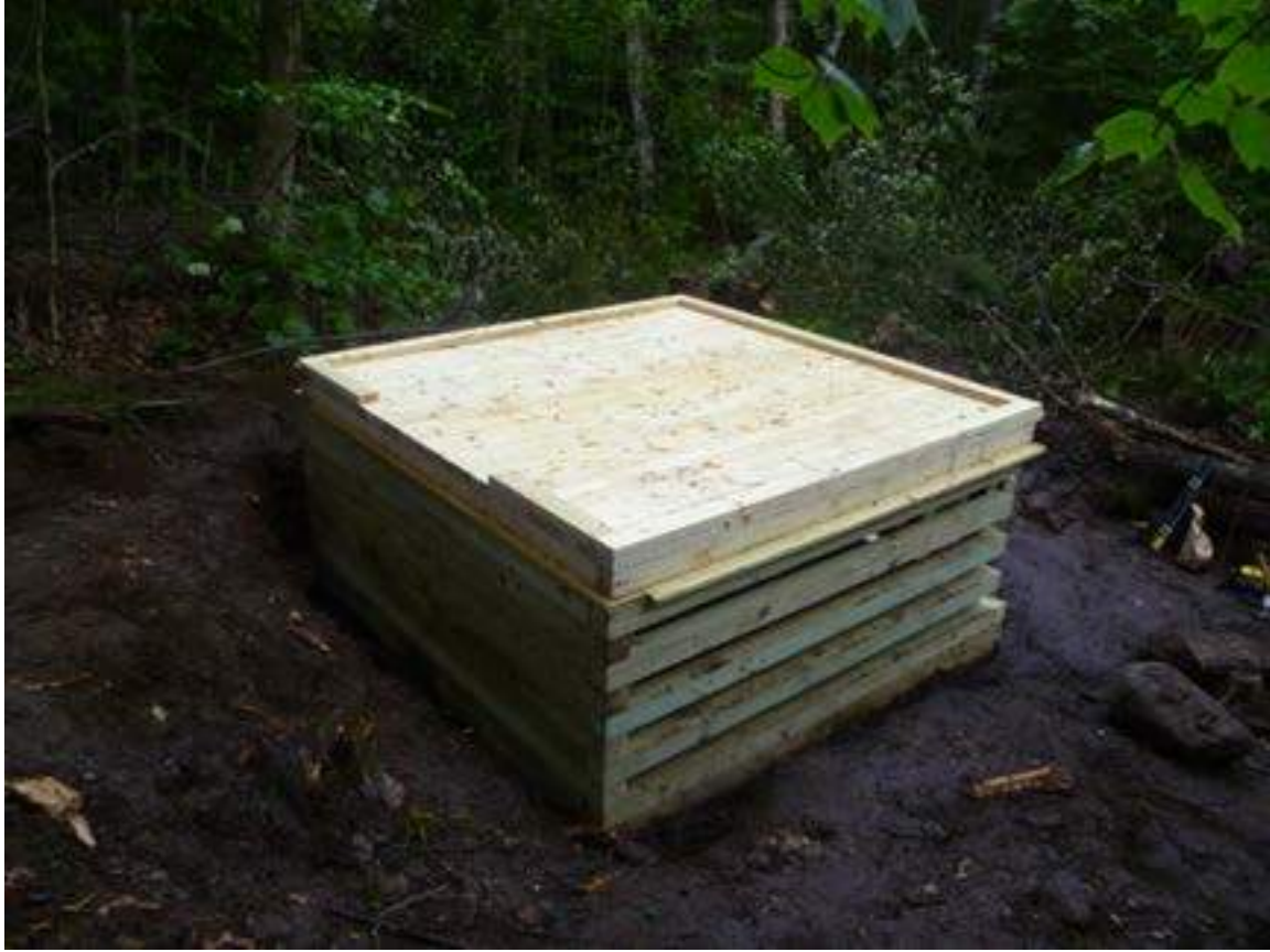
Completed floor and sill.
