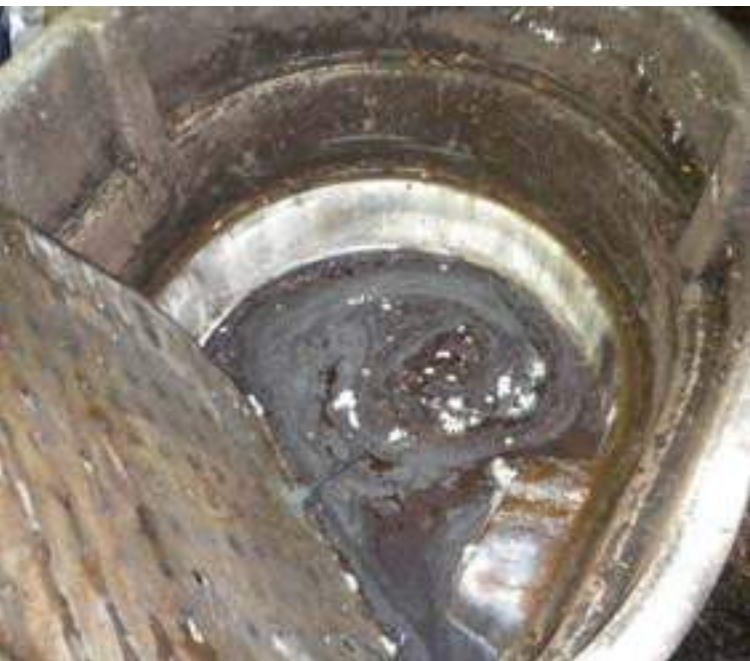
Strain Plate Removed
