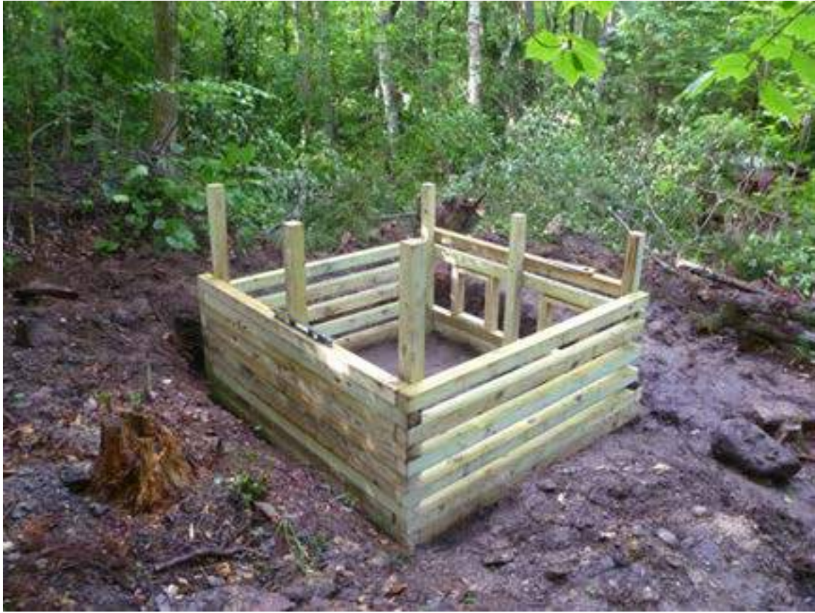
The completed moldering bin and six posts.
