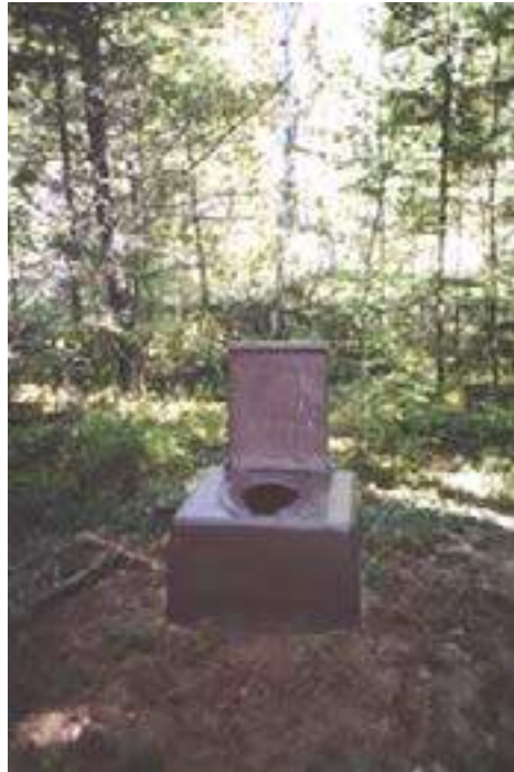
Figure 84—A fiberglass riser for a pit toilet in the Boundary Waters Canoe Area.
