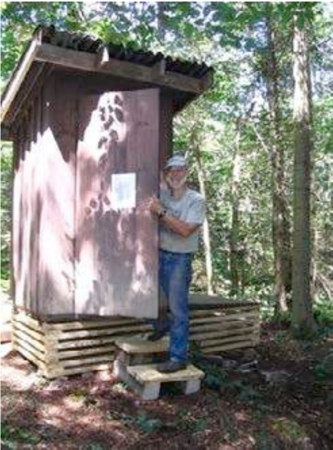
Photo #5. Project completed.
