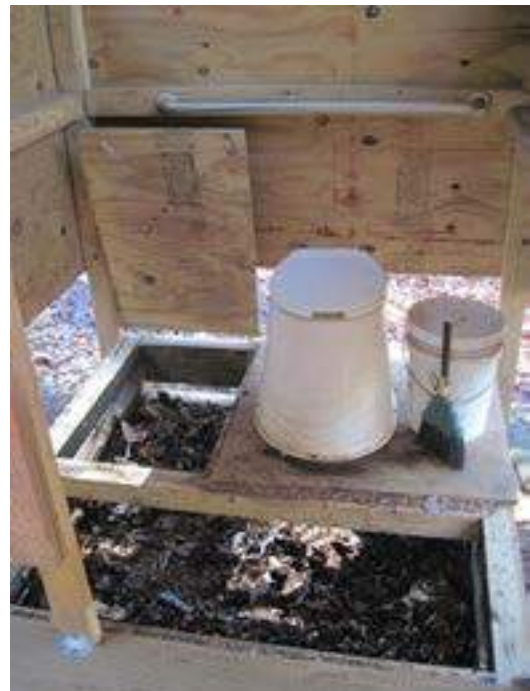
Two access doors allow for easy and sanitary leveling of the waste pile
