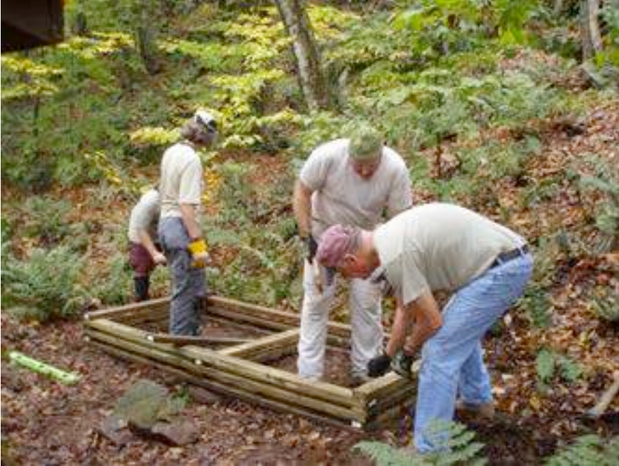
Photo #2. Crib assembly has begun.
