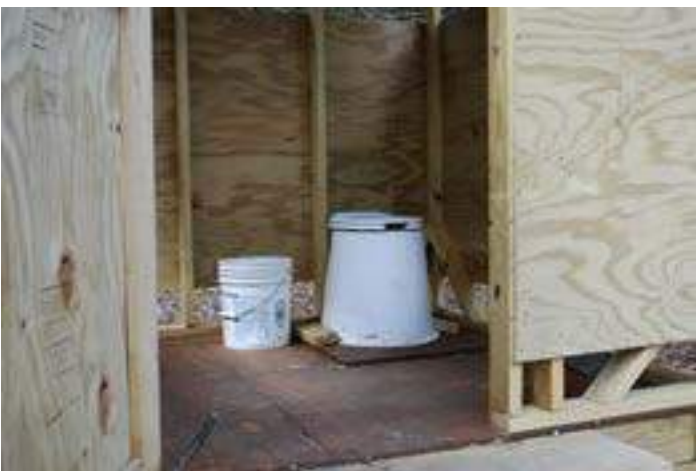
Interior of accessible Privy
