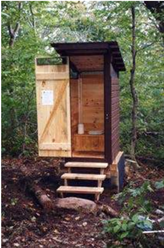
Non-Accessible Moldering Privy
