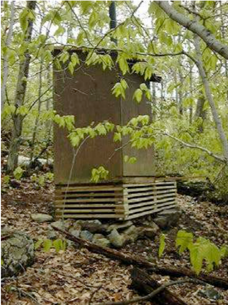
Photo 1. Crib set on rocks to compensate for sloping site.
