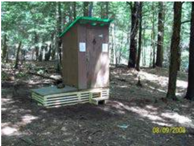
Completed Mass AMC Moldering Privy
