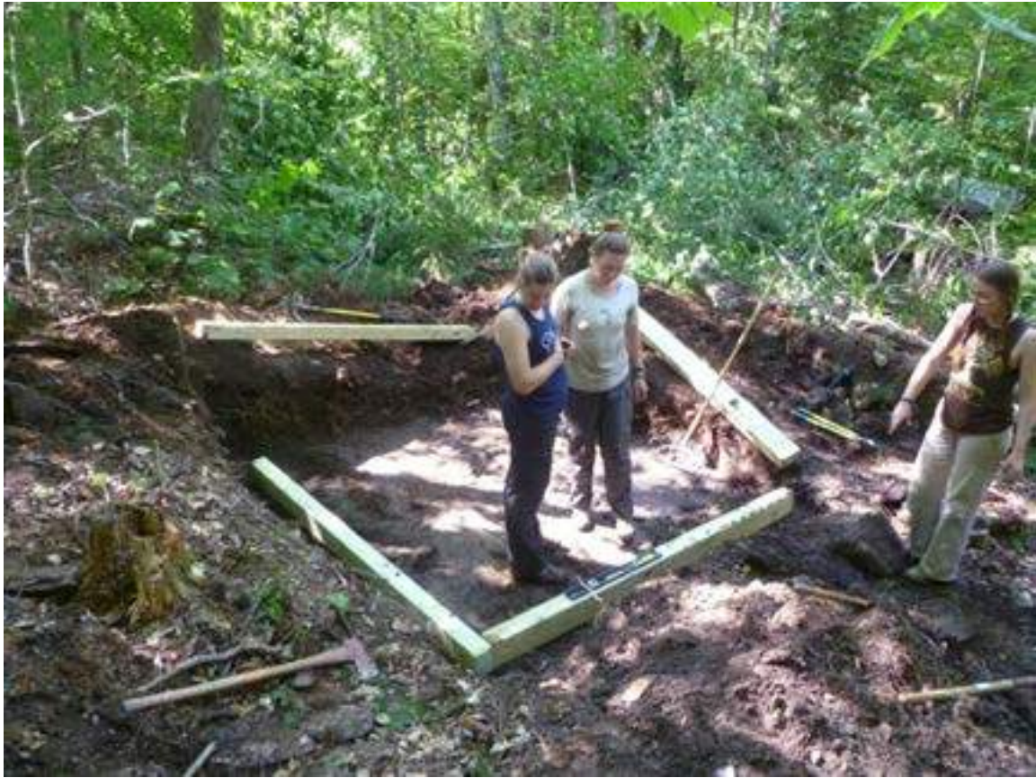
After digging out the site for the molding bin.
