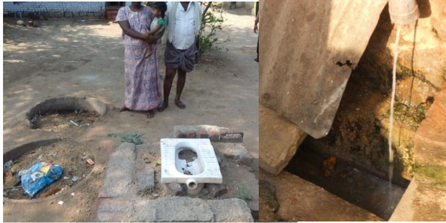
Dysfunctional pit latrines
